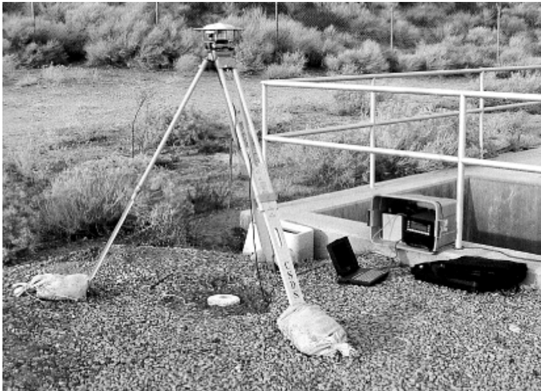
Figure 31. Temporary Global Positioning System (GPS) base station at the Antelope Valley–East Kern (AVEK) Water Agency district office in Antelope Valley, California.
