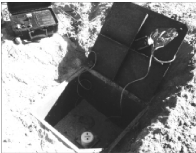
Figure 35. Typical tiltmeter installation for recording the magnitude and direction of ground tilting associated with direct well injection at Lancaster, Antelope Valley, California.
