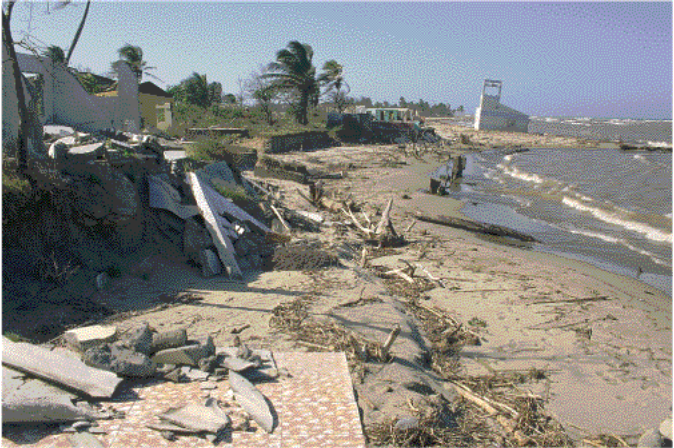
Figure 5. Houses destroyed by storm-surge wave action at Santa Rosa de Aguán, Honduras, during Hurricane Mitch.
