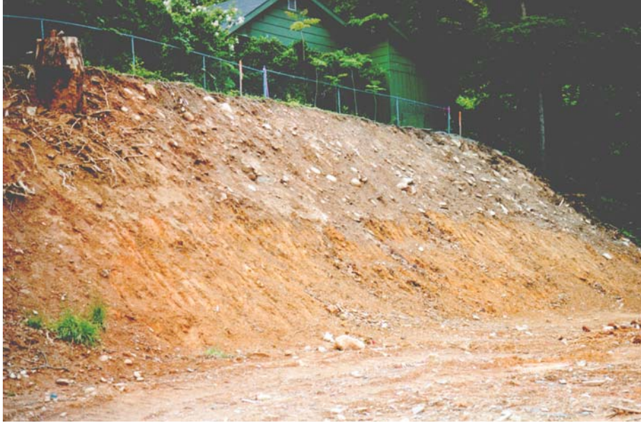
Fig. 10- Fluvial terraces have incised the boulder debris fan along Le Conte Creek on the lower part of the fan (elevation = 1400 ft). This excavation of a parking lot shows rounded cobbles of Thunderhead Sandstone deposited unconformably above weathered Roaring Fork Sandstone. The fence and house are approximately 100 ft above Le Conte Creek. This view is to the south, up the fan.
