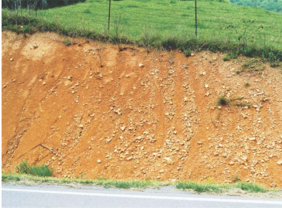
Fig. 23- Road cut, about 2 m high, in Wear Cove showing sub-rounded pebbles and cobbles of quartz in a red clay residuum derived from the weathering of Ordovician Limestone (elevation 1450 ft, Wear Cove quadrangle).
