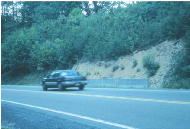
C) Landslide along Rt. 321, east of Gatlinburg in the Pigeon Siltstone.
