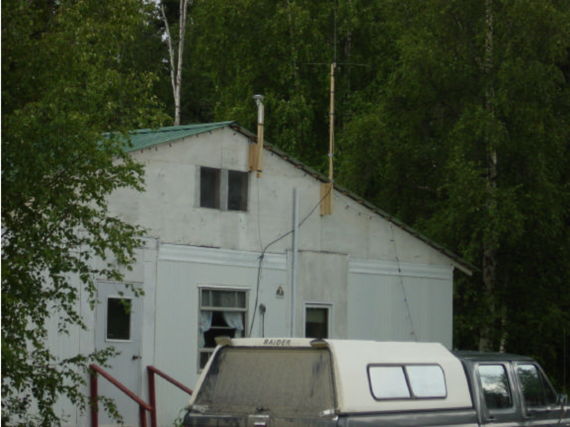
Illustration – Base Station GPS Antenna and Radio Modem Link
