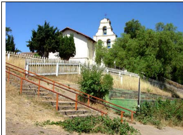
Figure 2-8. The San Juan Bautista Mission. The trace of the San Andreas Fault runs along the foot of a historic grandstand (painted green) along the "El Camino Real" (at the base of the stairs). The historic road runs along the San Andreas Fault scarp through the northeast side of town.
