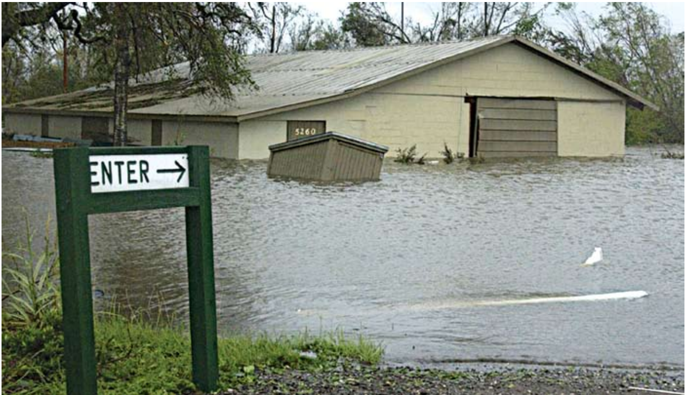
Figure 9. High water flooded structures near Blackwater River in Milton. Photo courtesy Pensacola News Journal, Copyright 2004.
