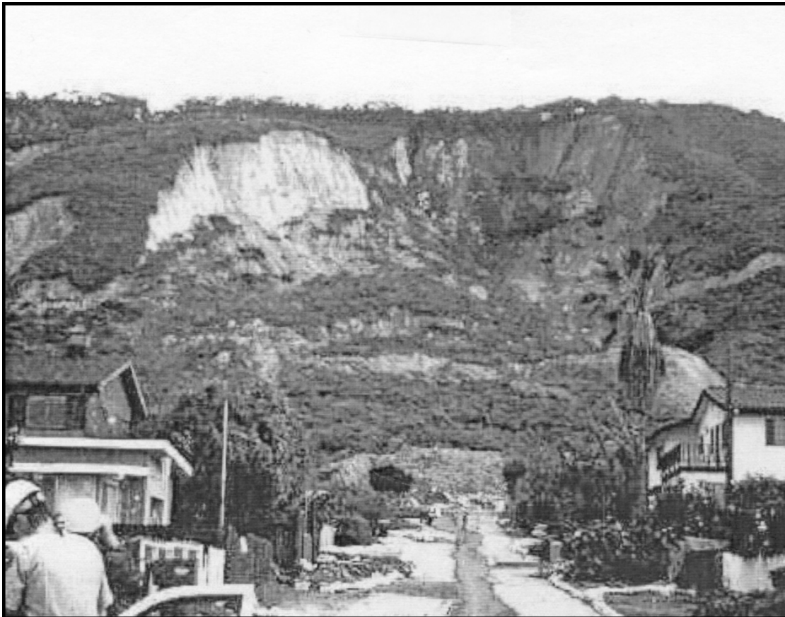
Photo 1: La Conchita Landslide: which buried six homes and destroyed three others on March 4, 1995 in Ventura County.
