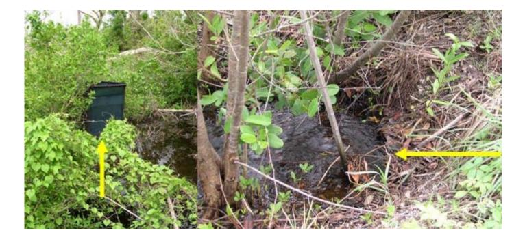
Figure 42. Water control structures along Powerline Road, Sanibel, Island, Florida. A structure (left, yellow arrow) on east side of the road that directs surface water from south to north. A partially collapsed culvert (right, yellow arrow) with water flowing from the Shell Mound Trail area to east under Powerline Road.
