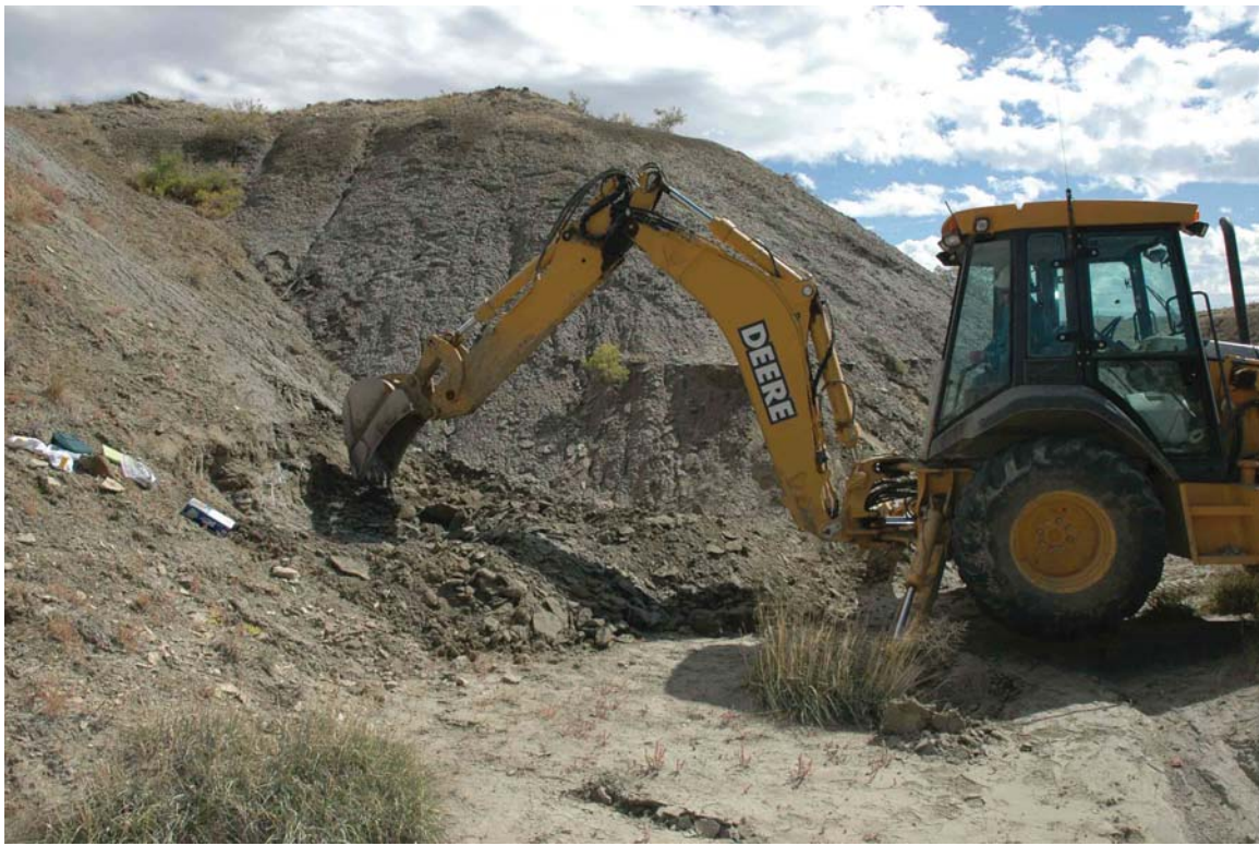
Figure 5. Backhoe excavating Fracture 1
