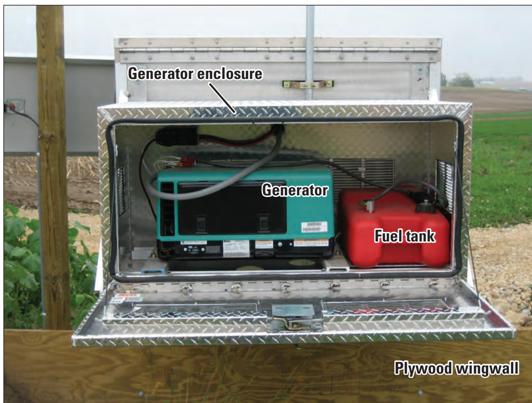
Figure 12. Remote-start generators were used to provide AC power at some stations.
