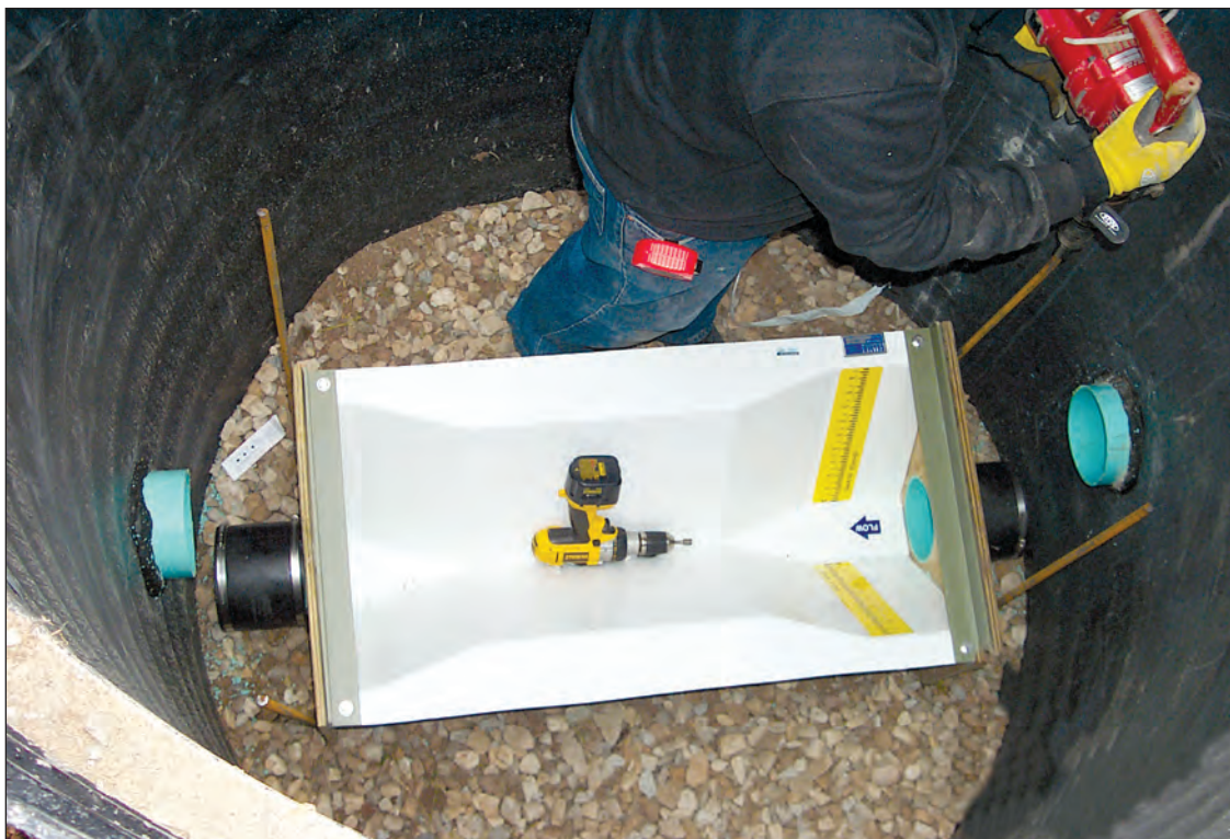
Figure 19. Extra-large, 60-degree, v-throat, trapezoidal flumes were installed inline with subsurface tiles within fields to compute discharge.
