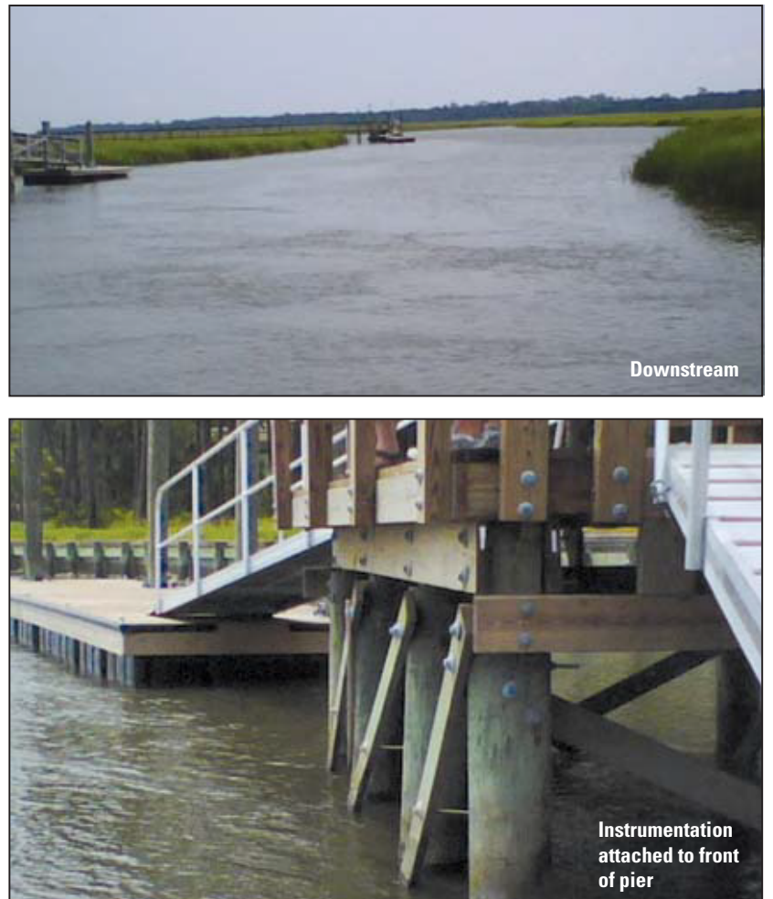
Figure 3. View downstream and of the public dock where the index-velocity instrumentation was attached on Cinder Creek.
