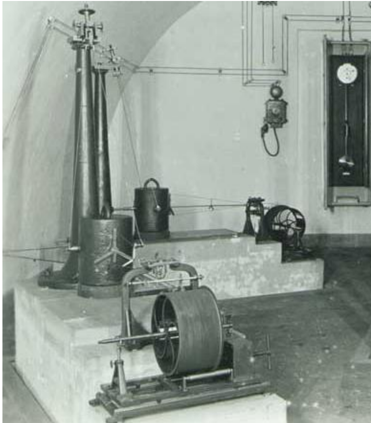
A Bosch-Omori seismograph like that in the Whitney Vault at HVO in 1933
