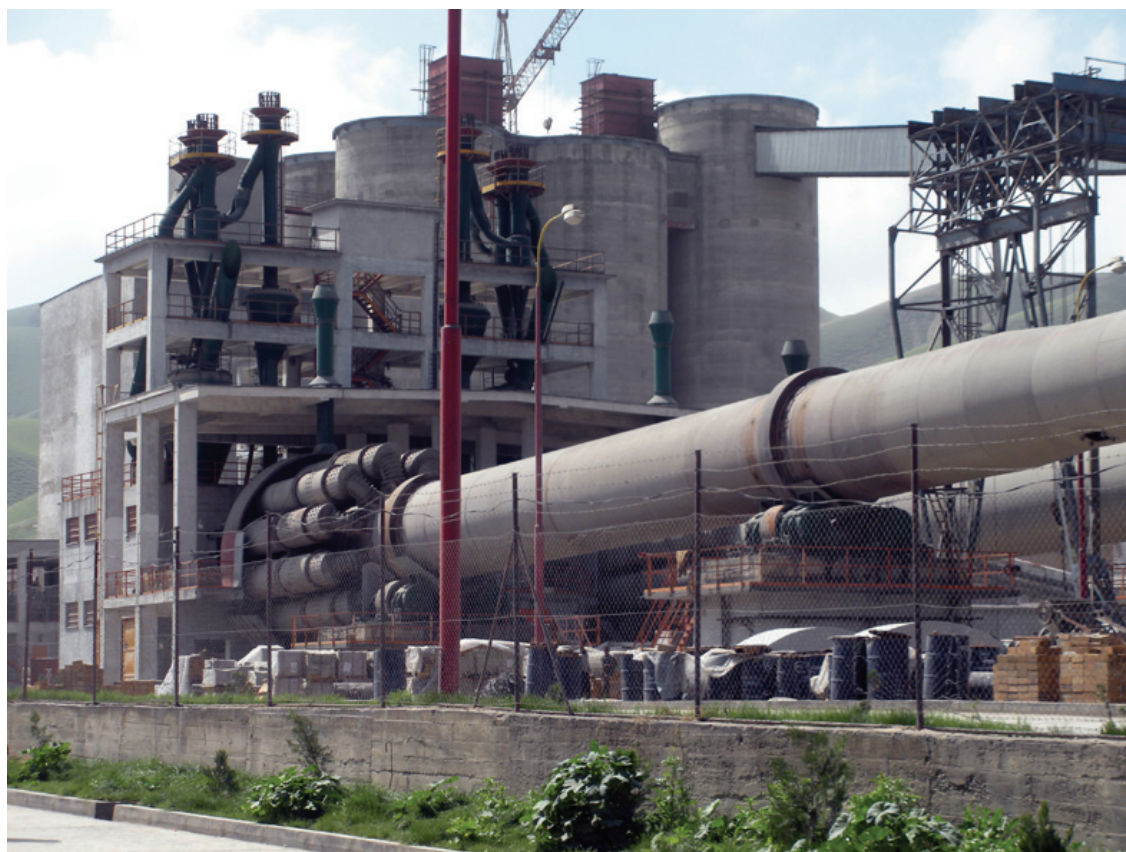
Figure 16B–16. View of the Ghorii II cement plant's 400-foot-long kilns and satellite coolers at Pul-e Khumri. Photograph by Victor G. Mossotti, U.S. Geological Survey.
