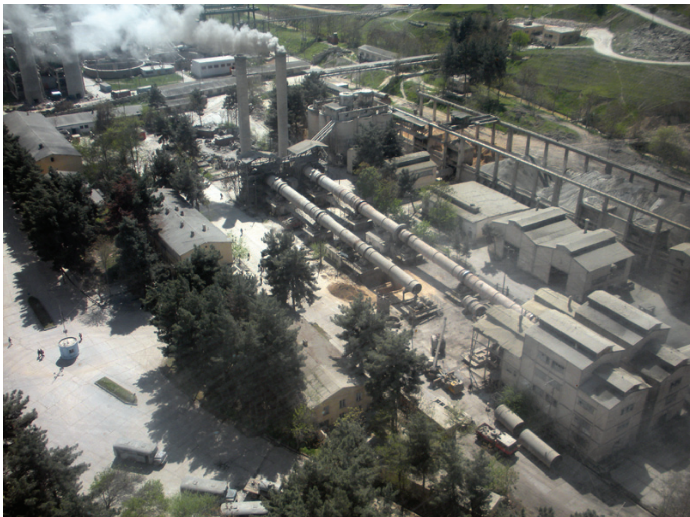
Figure 16B–13. View of the Ghorī I cement plant at Pul-e Khumri with kiln #2 dismantled for repair. Photograph by Victor G. Mossotti, U.S. Geological Survey.
