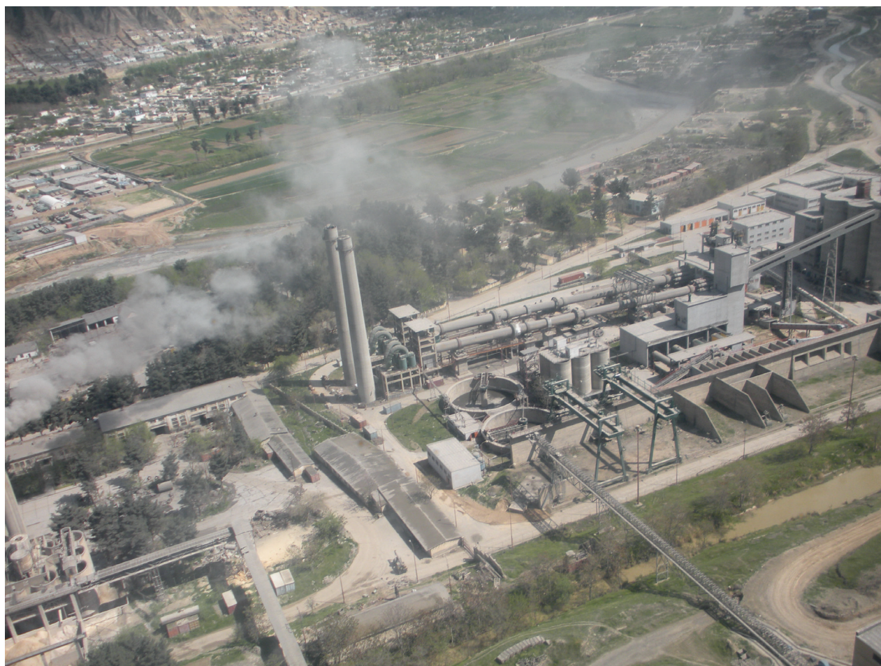
Figure 16B–15. View of the Ghorii II cement plant's dual 400-foot-long kilns. Photograph by Victor G. Mossotti, U.S. Geological Survey.
