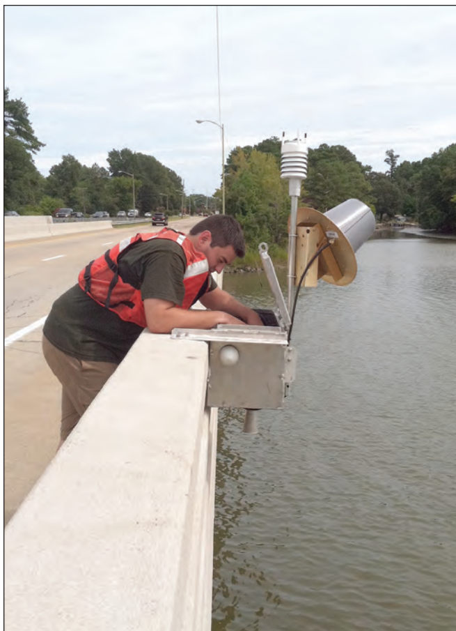
Figure 4. USGS employee installing rapid deployment real-time water-level gage at a site near Norfolk, Virginia (photograph by Andrew E. Knaak, USGS).
