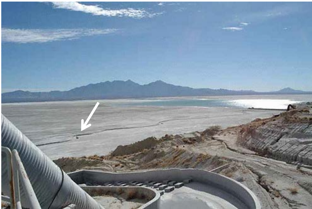
Figure 4. Photograph of the tailings storage facility for the Sierrita copper porphyry mine in Arizona. Note the slurry pipeline in the foreground and where it traverses the tailings as indicated by the white arrow. The sun's reflection can be seen on the tailings pond in the right-middle portion of the photograph. Photograph courtesy of Freeport-McMoRan Copper & Gold Inc.; used with permission.
