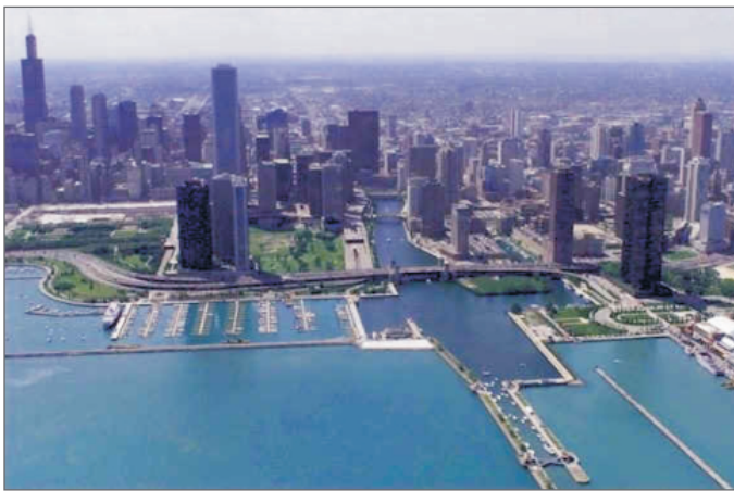
Figure 5. The Chicago River Controlling Works, Chicago Lock, and DuSable Harbor, Chicago, Illinois.
