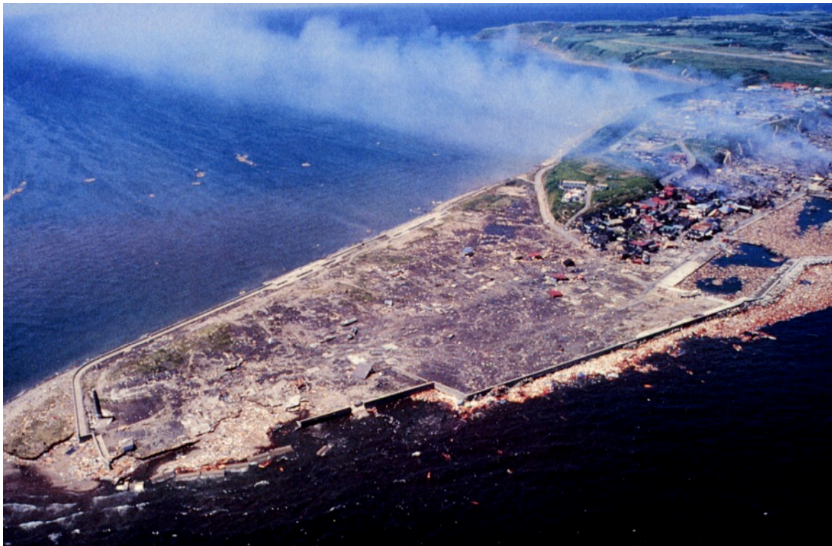
Figure 80. Photograph of fire ignitions in the town of Aonae on the southern tip of Okushiri Island, Japan, following the 1993 Hokkaido Nansei-oki earthquake and tsunami (photograph from Yanev and others, 1993).
