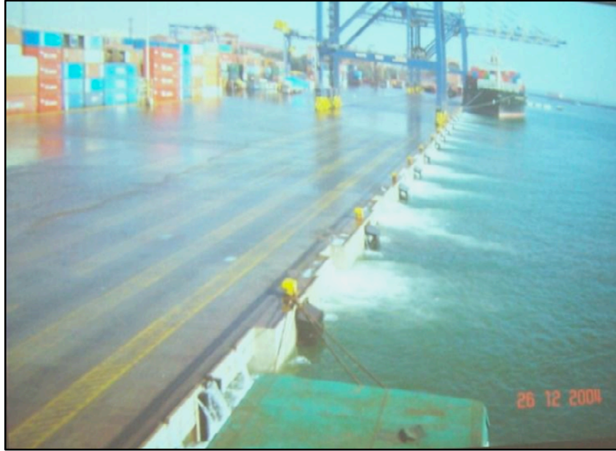
Figure 13. Photograph of flooding of container wharf at Port of Chennai, India, in the 2004 Sumatra Tsunami (4.1-meter tsunami wave) (photograph by Martin Eskijian).
