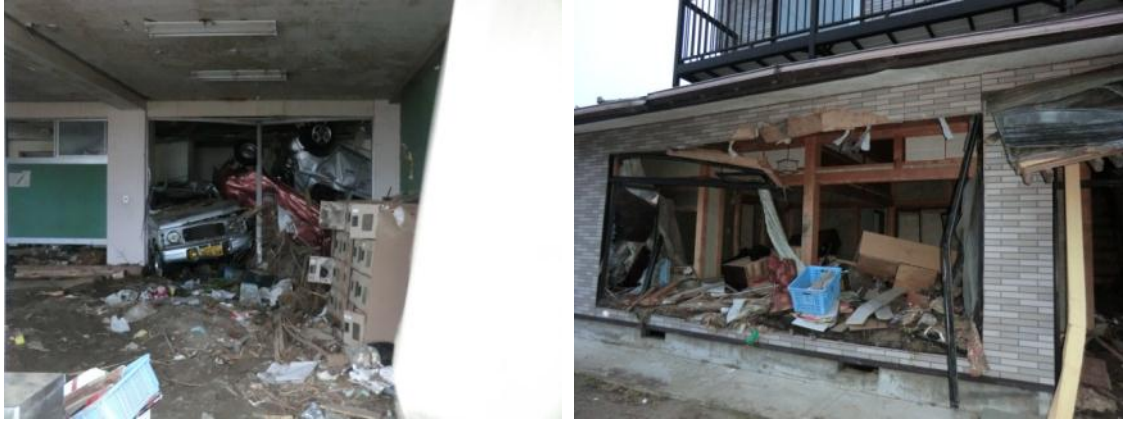
Figure 57. Photographs of wetting, soiling, and deposition of debris in buildings in Japan affected by the 2011 Tohoku tsunami (photographs by Keith Porter).
