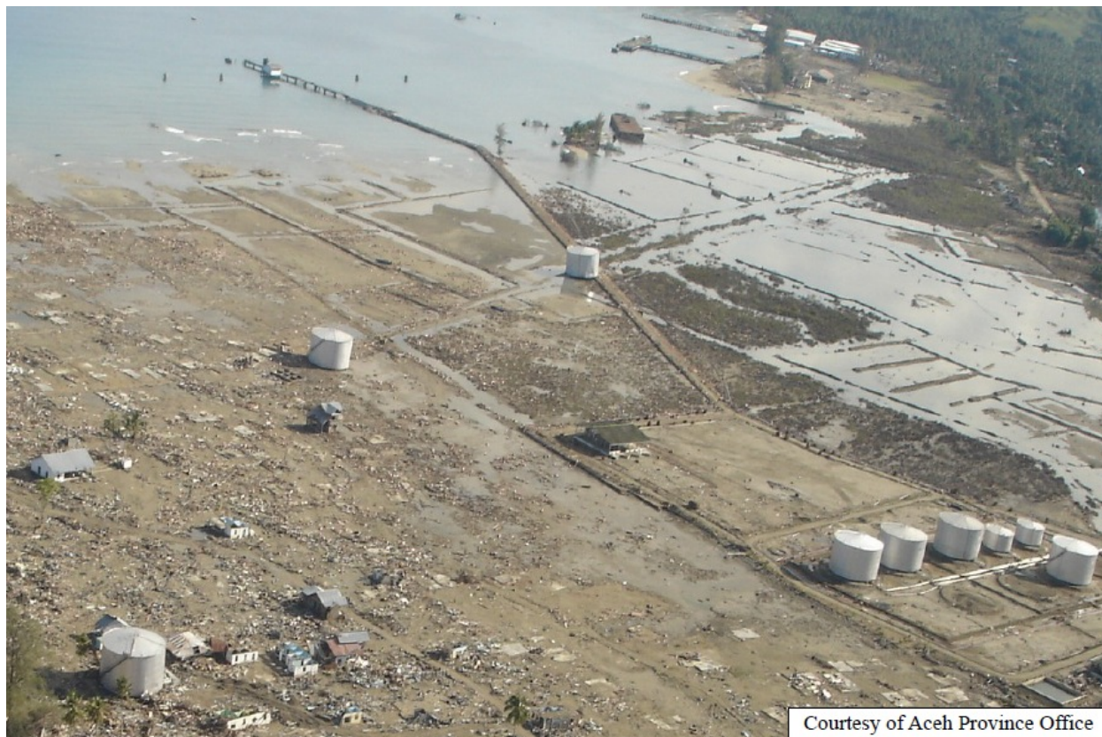
Figure 83. Photograph of Krueng Raya, Aceh, Indonesia, deep water port after the 2004 Indian Ocean tsunami. Three tanks (reported to have been empty or near empty) of nine tanks floated about 500 meters. (Photograph from Aceh Province Office.)
