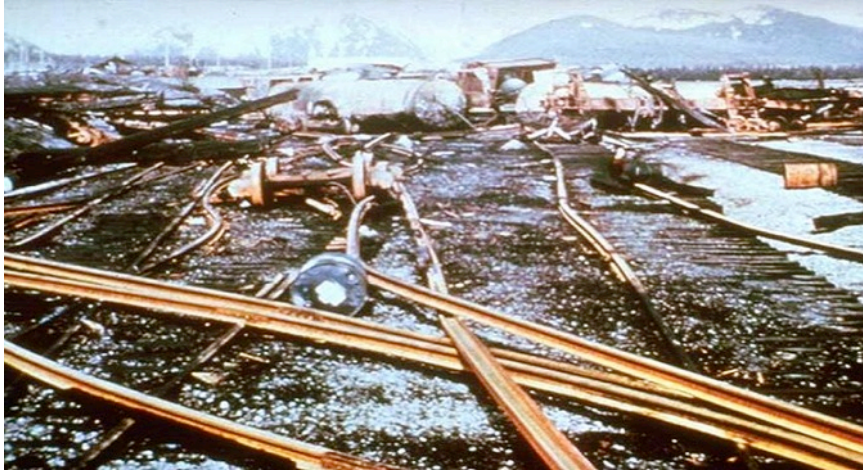
Figure 73. Photograph of Seward yard after 1964 Alaska tsunami. Estimated wave height in the Seward yard is between 25 and 35 feet (photograph courtesy of National Oceanic and Atmospheric Administration, National Geophysical Data Center).
