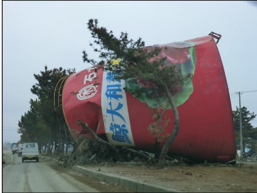
Figure 23. Photograph of tank floated off its foundation during the 2011 Tohoku, Japan, tsunami (photograph by Keith Porter).
