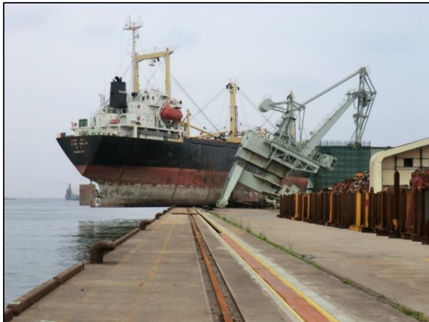
Figure 3. Photograph of MV Glovis Mercury displaced on top of wharf and damaged crane at Sendai Port, Japan, during 2011 Tohoku tsunami (photograph by Keith Porter).
