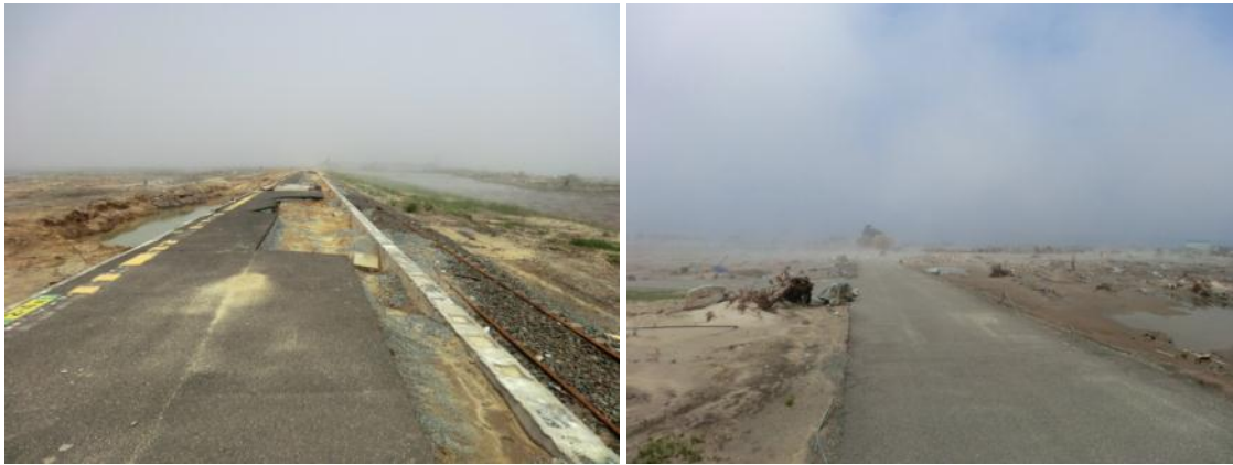
Figure 62. Photographs showing a contrast in tsunami scour potential resulting from roadway elevation. The left image is a view looking north from a commuter railway platform on the Sendai, Japan, plain. Before the 2011 Tohoku tsunami, it had had rail on both sides of the platform; now only a short stretch on the east (ocean) side and large scour pits on the west (landward) side. There is no sign of the railbed or rail. On the right is a nearby road, largely undamaged, on the seaward side of the rail line. The road is largely undamaged. (Photographs by Keith Porter.)
