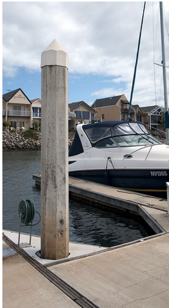
Figure 50. Photograph of a concrete dock piling (from Wikimedia Commons).
