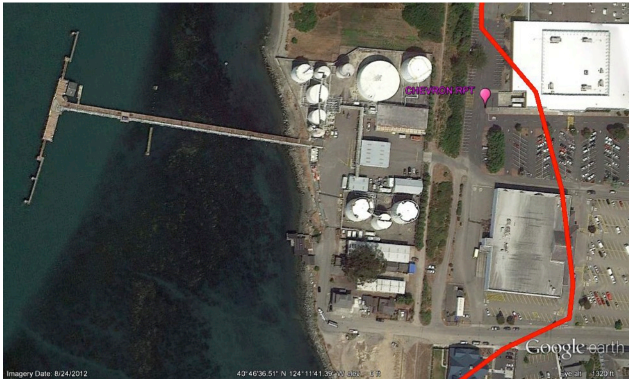
Figure 90. Satellite image of a Humboldt Bay, California, oil facility. In this image the approximate extent of inundation as determined by others in this report is shown by the red line (base image from Google Earth).
