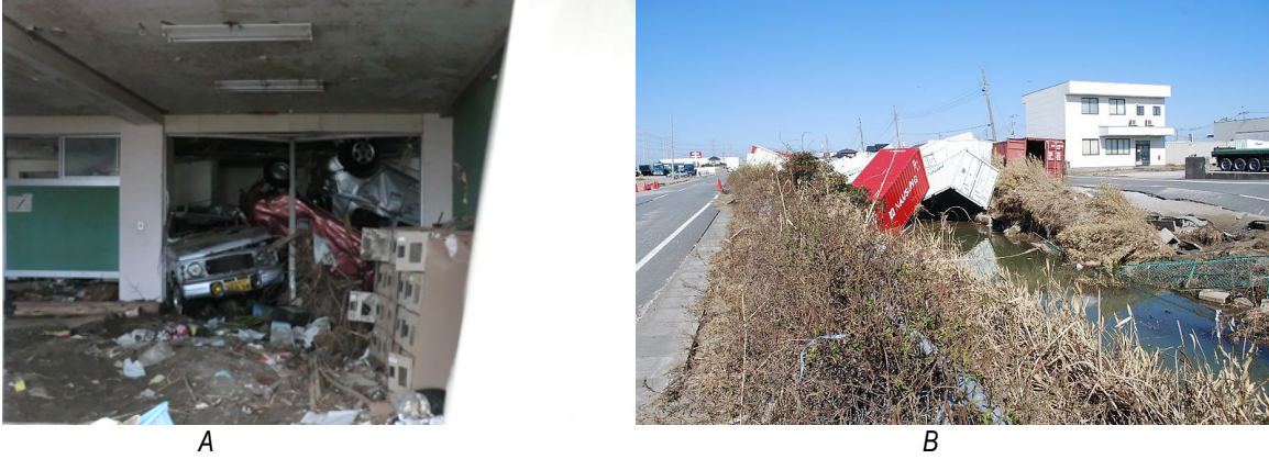
Figure 19. Photographs of damage by the 2011 Tohoku, Japan, tsunami. A , Cars floated into a building by the 2011 Tohoku tsunami (photograph by Keith Porter). B , Cargo containers in Kashima after the 2011 Tohoku tsunami (photograph from Wikimedia Commons).
