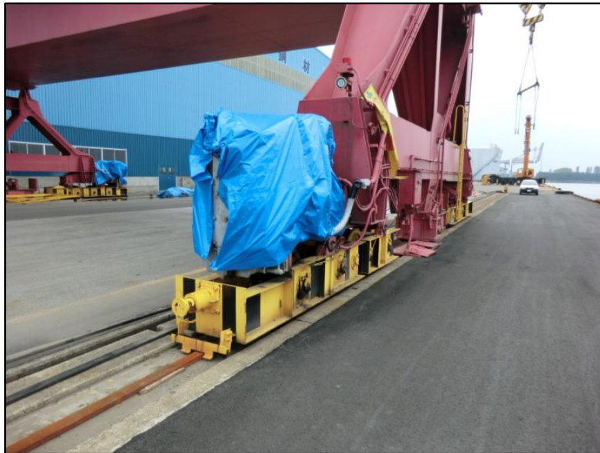
Figure 14. Photograph of damaged container crane motor in Port of Sendai, Japan, following the 2011 Tohoku tsunami (photograph by Keith Porter).
