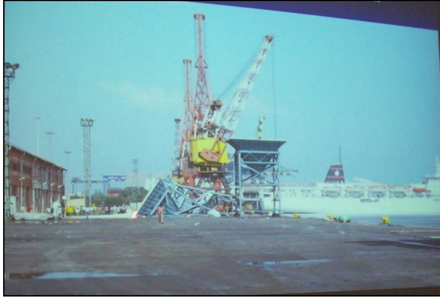
Figure 8. Photograph of hoppers destroyed by out of control vessel in Port of Chennai, India, during the 2004 Sumatra Tsunami (photograph by Martin Eskijian).
