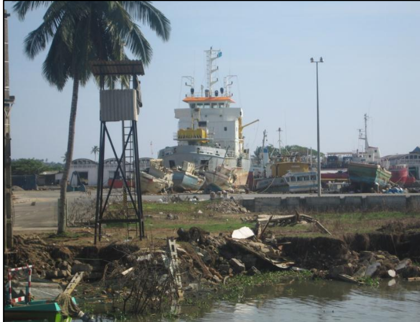
Figure 2. Photograph of Sri Lanka Port of Galle dredge grounded on wharf by a 5.3-meter tsunami wave during the 2004 Sumatra tsunami (photograph from American Society of Civil Engineers, Coasts, Oceans, Ports, and Rivers Institute, 2005).
