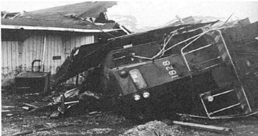
Figure 72. Photograph of overturned locomotive at Seward after 1964 Alaska tsunami. Run-up height at Seward after the 1964 Alaska tsunami was about 40 feet. (Photograph from Sturman, 1973.)
