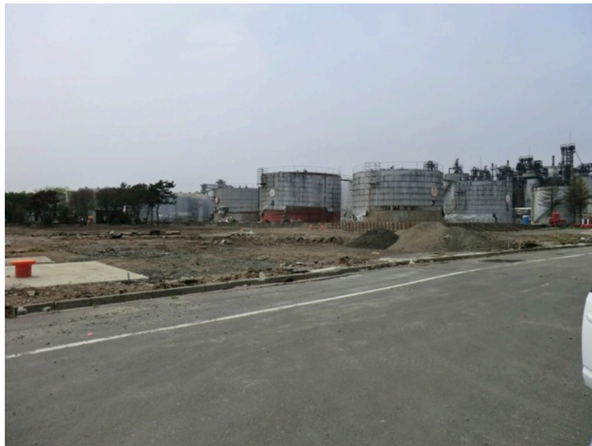
Figure 22. Photograph of tsunami-damaged tanks in Ishinomaki, Japan, after the Tohoku 2011 tsunami (photograph by Keith Porter).
