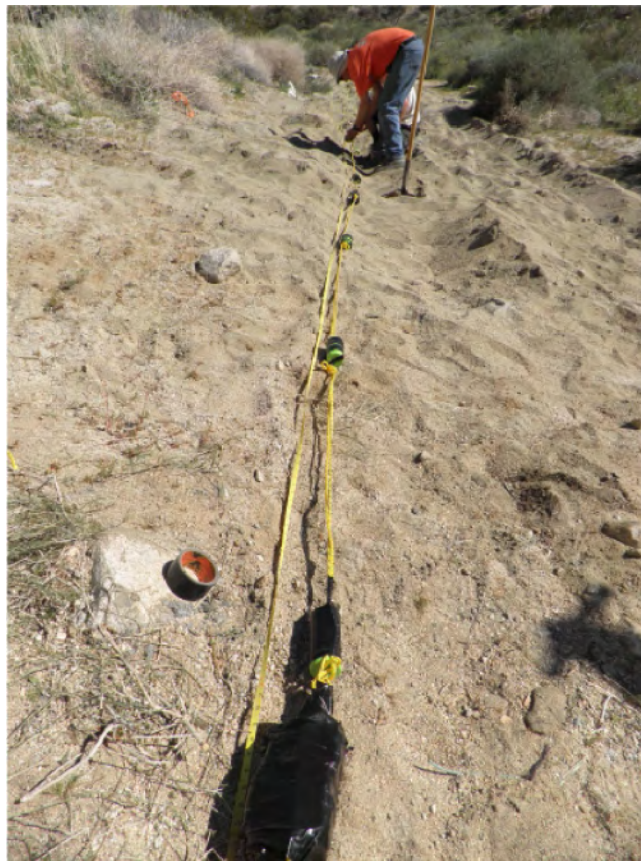
Figure 12. Photograph of detonating cord and booster assembly. Boosters (green cylinders) were threaded onto and taped securely to the detonating cord (yellow) at fixed intervals (measuring tape shown on left side of the assembly). A brick (or rock), seen at the bottom of the photograph, was taped onto the bottom of the assembly to prevent assembly from floating upward during pumping of blasting agent into the shot hole.
