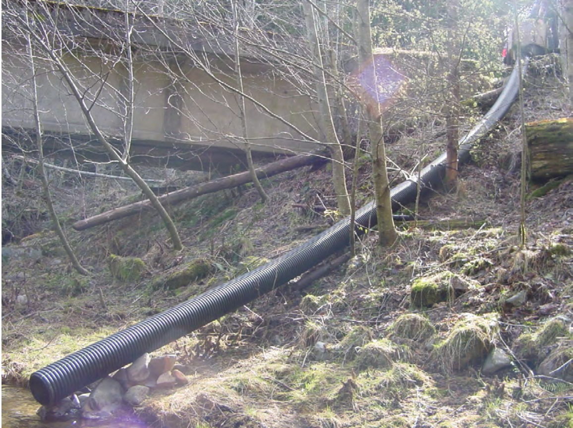
Figure 2. Photograph showing release pipe used by trap-and-haul staff to release adult coho salmon ( O. kisutch ) and steelhead ( O. mykiss ) in Hoffstadt Creek, Washington.
