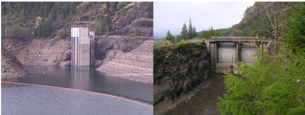
Figure 1. Photographs showing forebay and water passage structures at Cougar Dam, Oregon. Left photograph shows earthen dam, cul-de-sac, and temperature control tower at western end of dam. Right photograph shows spillway Tainter gates at eastern side of the dam. Photographs taken by John Beeman, U.S. Geological Survey, November 16, 2010, during reservoir elevation of 1,580 feet.
