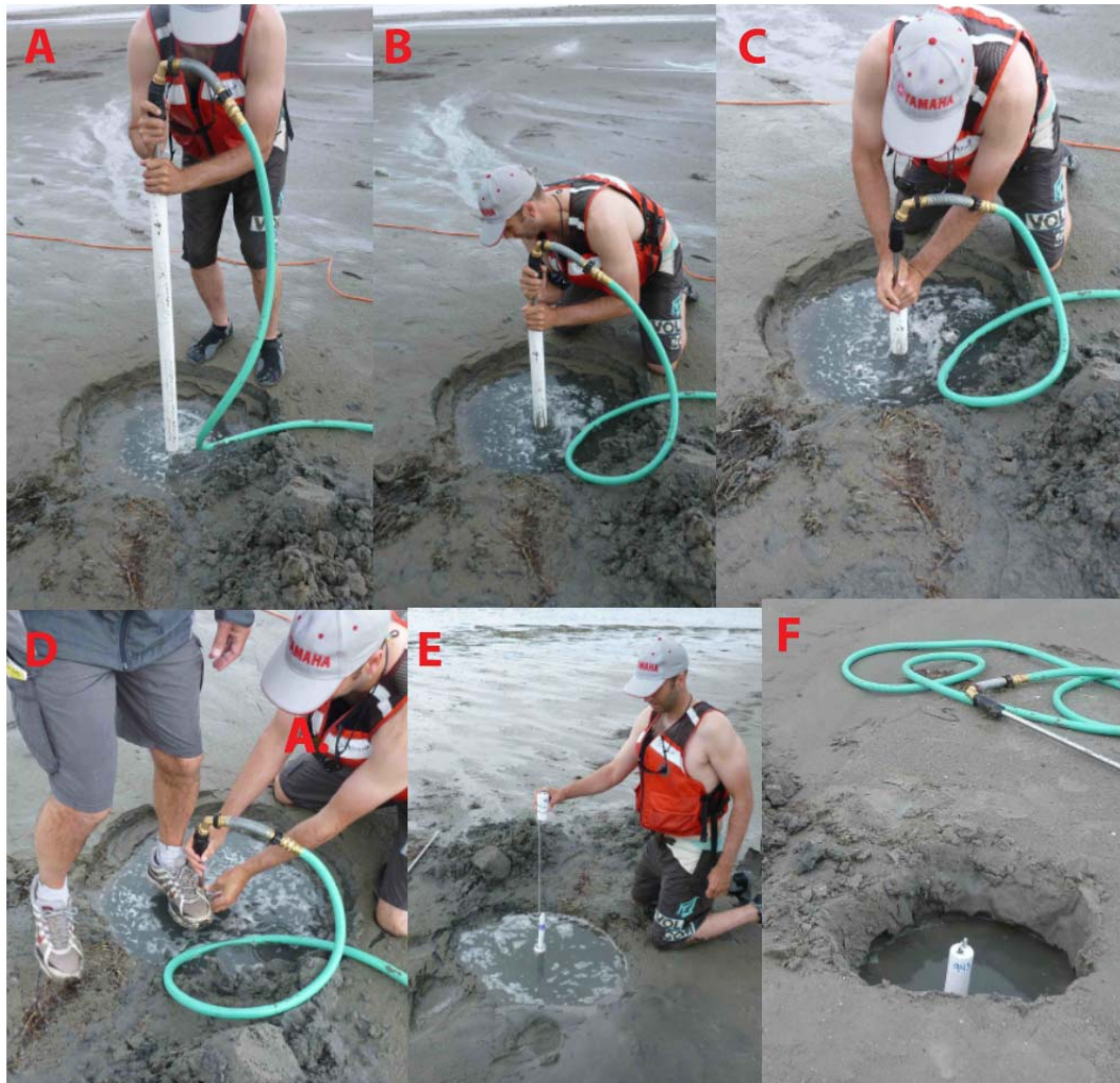
Figure 5. Photographs illustrating the procedure for the installation of a buried well on Dauphin Island, Alabama, in 2013. A–C , well casing being jetted into the sand; D , well casing at the end of jetting; E , pressure sensor inserted into the casing; and F , completed installation with pressure sensor inserted and cap screwed into the well casing.
