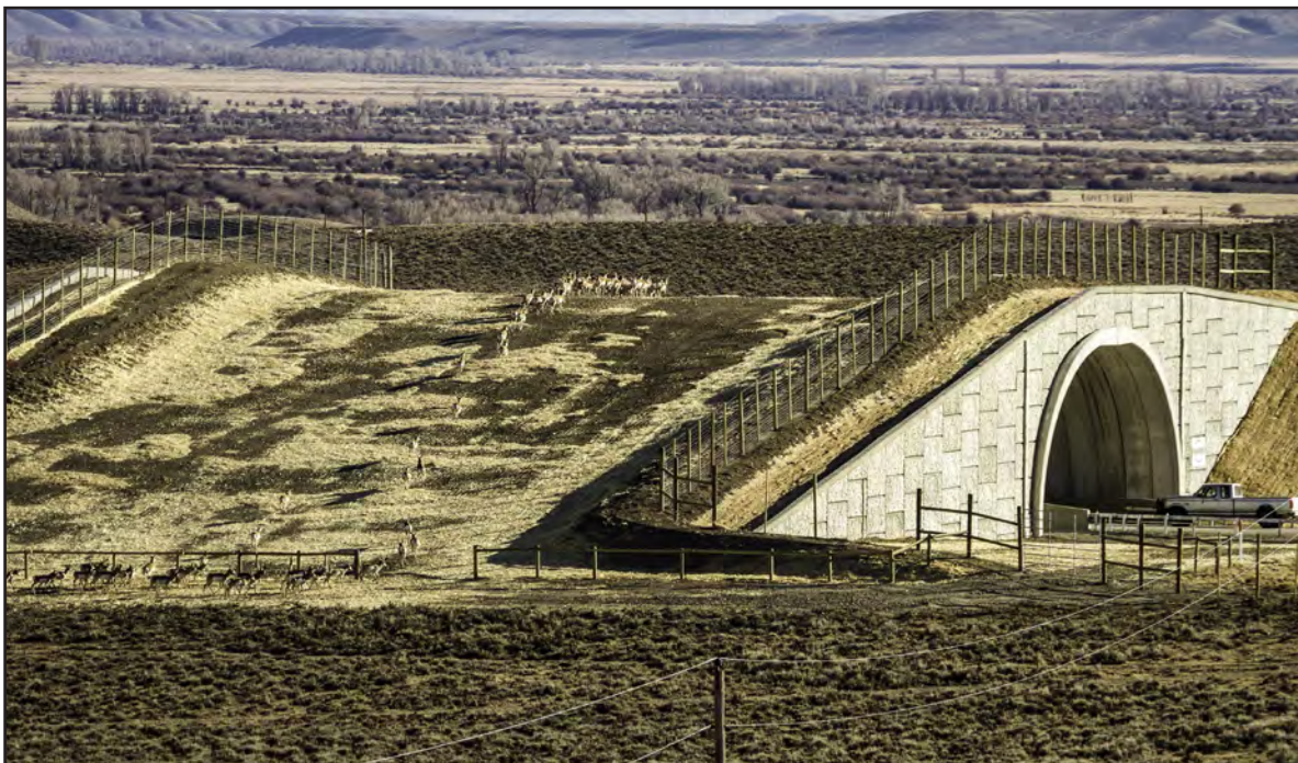
Figure 2–5. Pronghorn ( Antilocapra americana ) make use of a wildlife highway overpass at Trappers Point, Wyoming (Photograph by Jeff Burrell, Wildlife Conservation Society).
