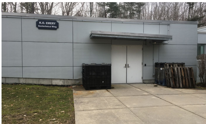
Figure 2. The K.O. Emery Geotechnical Wing of the U.S. Geological Survey offices in Woods Hole, Massachusetts (2018). Photograph by Brian Buczkowski, U.S. Geological Survey.
