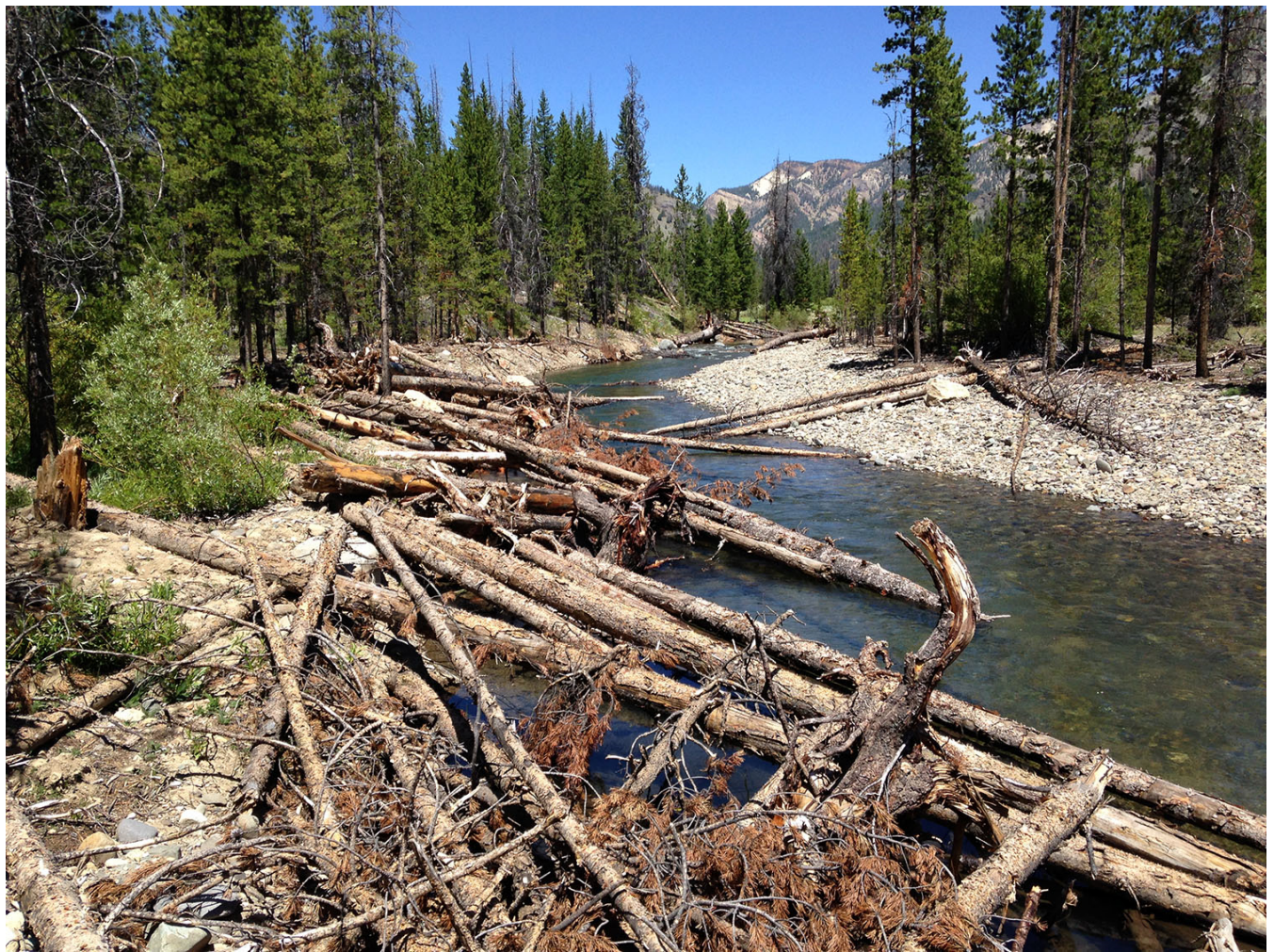
Figure 3. Photograph showing engineered log jams on the Yankee Fork of the Salmon River near Stanley, Idaho. Photograph by Bureau of Reclamation, date unknown.
