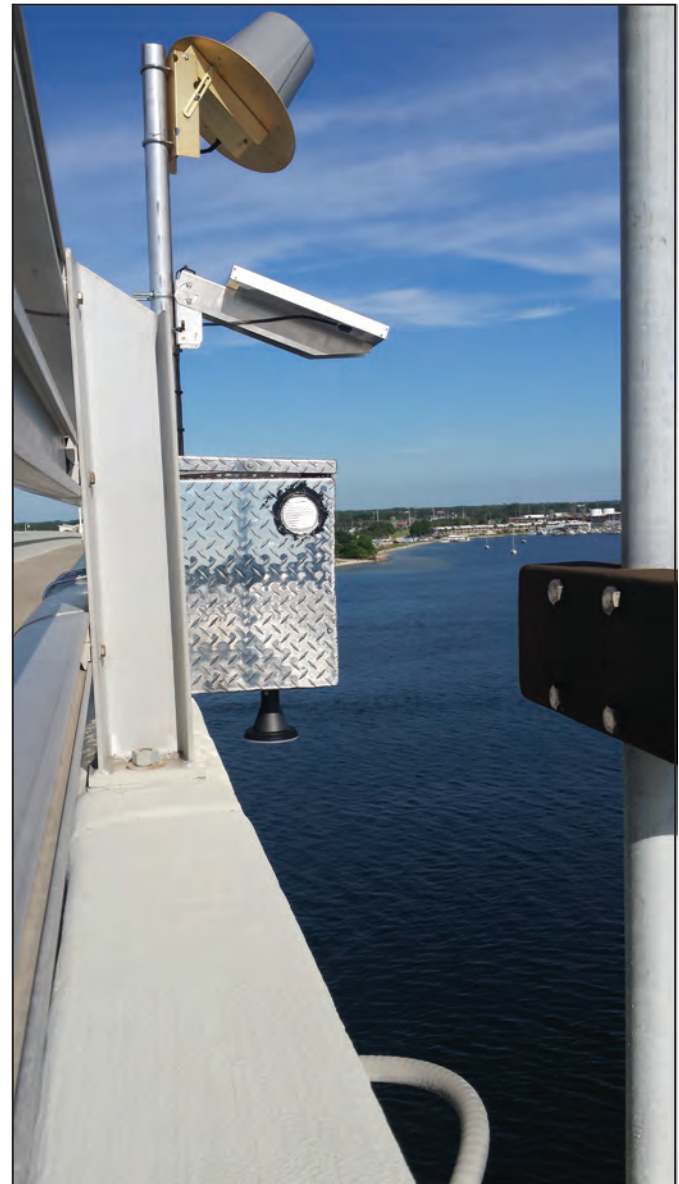
Figure 4. U.S. Geological Survey (USGS) rapid deployment gage collecting real-time water-level and barometric pressure data at U.S. Highway 98 in Panama City Beach, Florida, August 2015. Photograph by Mark Stephens, USGS.
