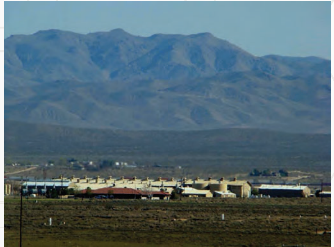
Figure 1. Pacific Gas and Electric Company (PG&E) compressor station, Hinkley, California, March 2009. (Photograph by Steven Perry, ARCADIS, Inc., courtesy of PG&E).
