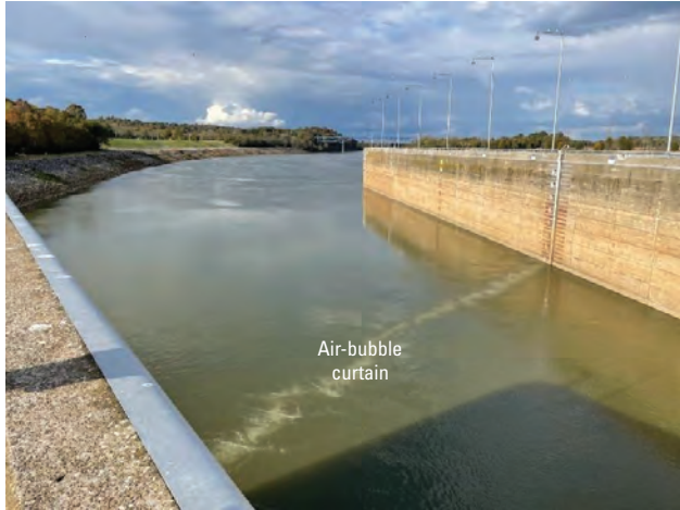
Figure 1. The multimodal deterrent system is installed in the downstream approach at Barkley Lock and Dam. The system, stretching across the width of the lock approach, consists of an air-bubble curtain, lights, and sound. Photograph by Andrea Fritts, U.S. Geological Survey.
