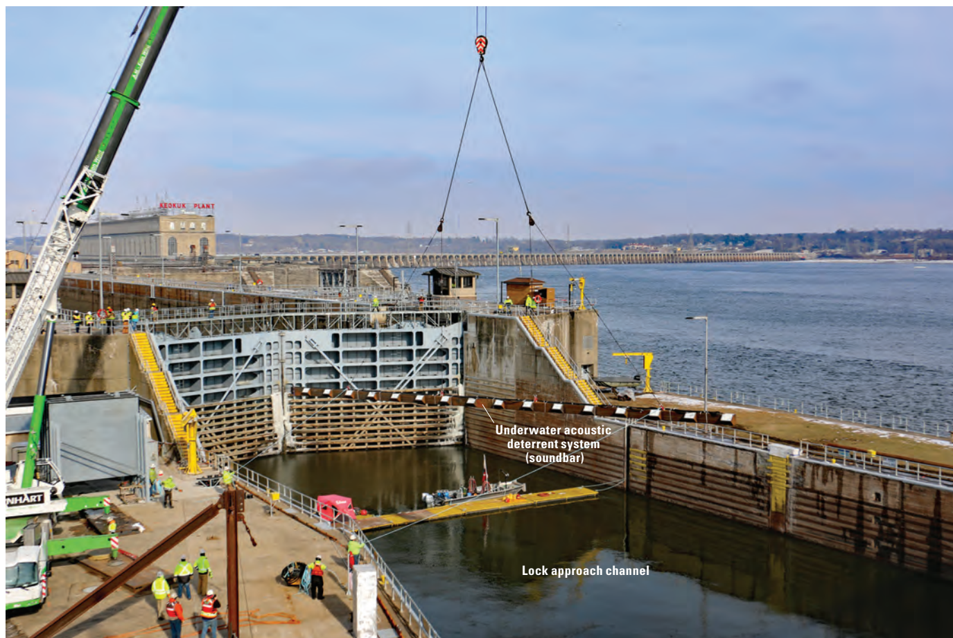
Figure 1. The underwater acoustic deterrent system being installed in the downstream lock approach channel of Mississippi River Lock 19, Keokuk, Iowa, in February 2021. Photograph by Mark Cornish, U.S. Army Corps of Engineers.
