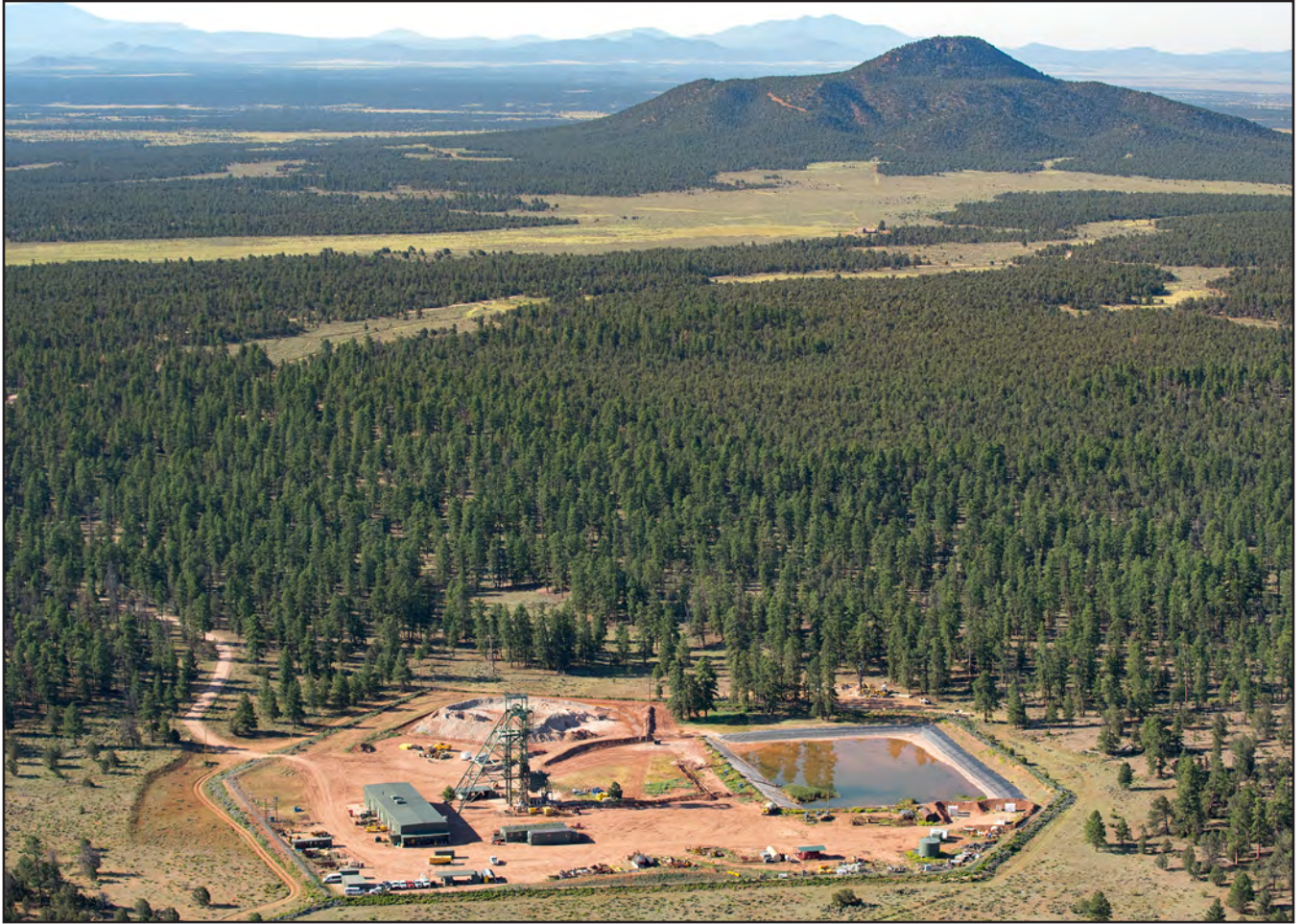
Figure 3. The Pinyon Plain mine (foreground) is located near Red Butte (near background) in Northern Arizona. Photograph by Blake McCord, freelance photographer.
