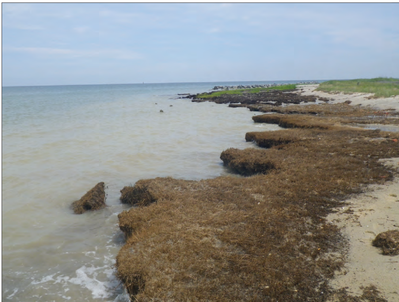
Figure 21. Wave-cut gullies along the low marsh edge in the embayment area of the Fog Point Living Shoreline Restoration Project site, July 2017. Photograph by Hongqing Wang, U.S. Geological Survey.
