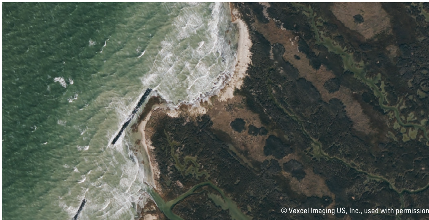
Figure 17. Wave overtopping at the breakwaters during November 23, 2020, storm surge (wave height was greater than 0.9 meter). Fringing low marsh Spartina alterniflora behind the structures was protected from wave impact. A low marsh zone in the embayment (gaps between segmented breakwaters) was inundated, however, and waves reached the sand berm line and high marsh ( S. patens ) zone. Image courtesy of Vexcel Imaging, used with permission.
