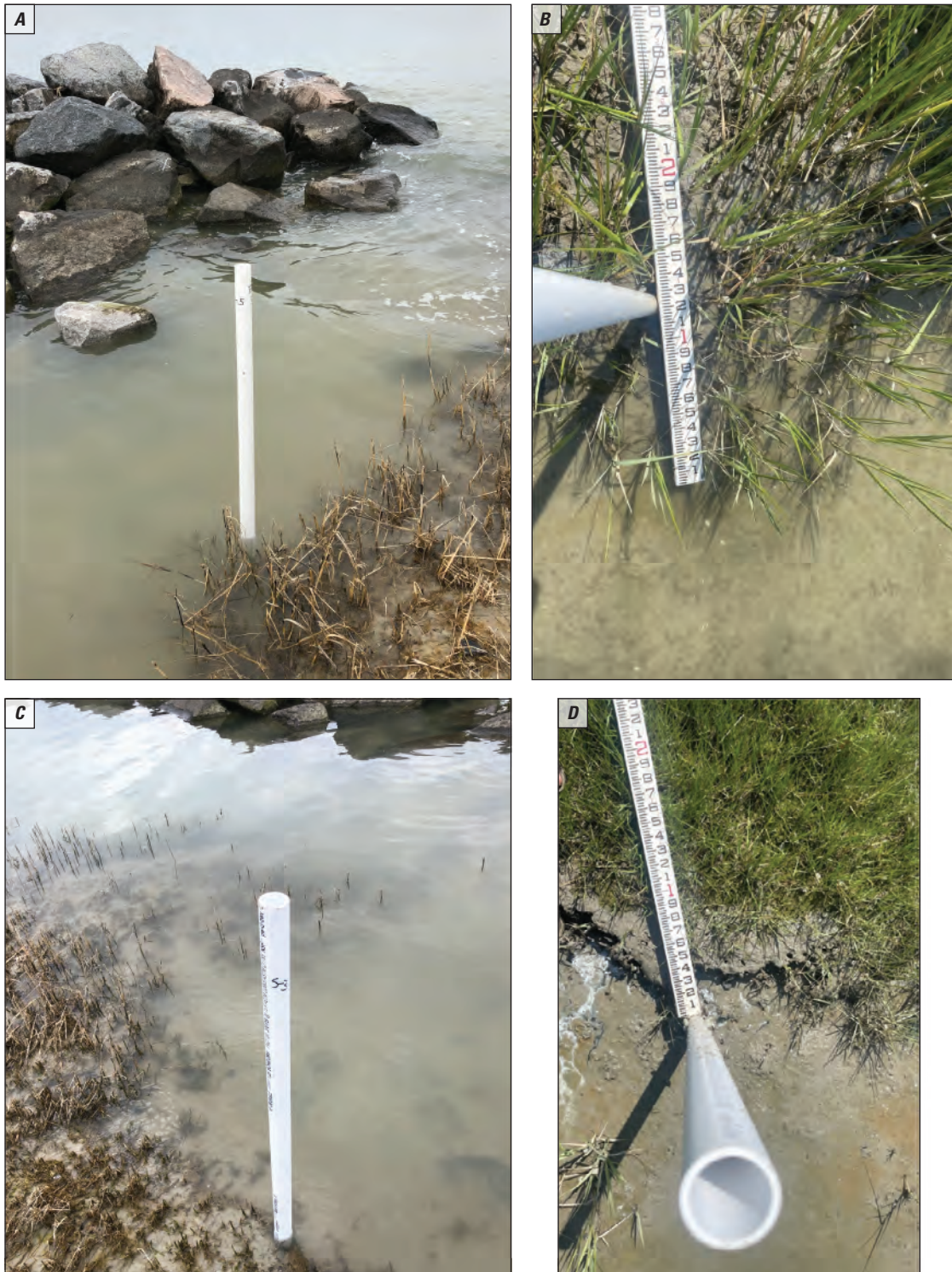
Figure 19. A and B , Lateral marsh accretion at Eps5 behind the breakwater during deployment in February 2020 and C and D , erosion at Eps3 behind the breakwater during retrieval in August 2021 at the Fog Point Living Shoreline Restoration Project site in the Glenn Martin National Wildlife Refuge, Maryland. Photograph A by Qin Chen, Northeastern University. Photographs B and D by William D. Capurso, U.S. Geological Survey. Photograph C by Hongqing Wang, U.S. Geological Survey.
