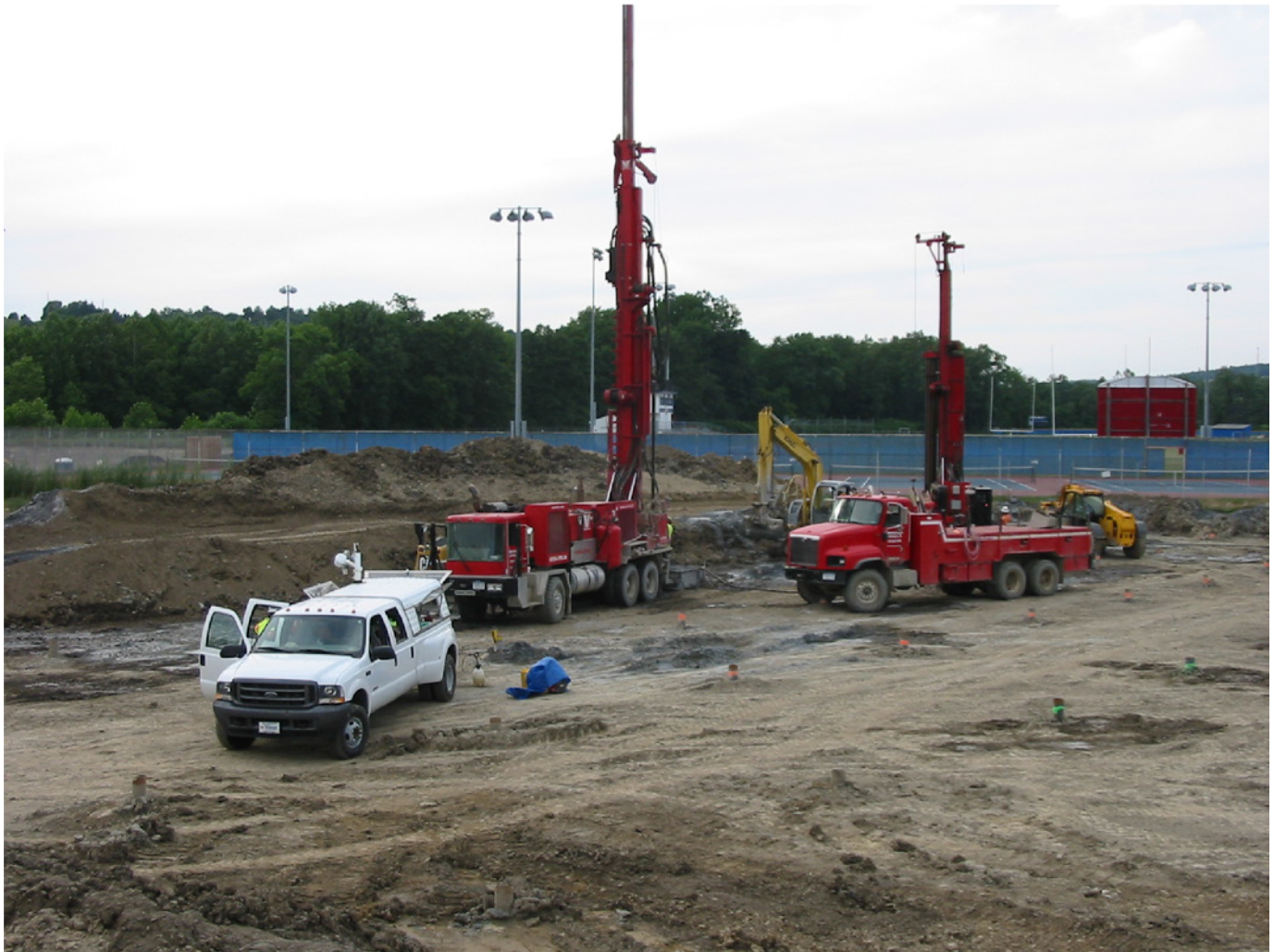
Figure 1. Photograph showing drilling rigs completing bores at the Owego-Apalachin Elementary School geothermal field, Tioga County, New York. Photograph by John H. Williams, U.S. Geological Survey.
