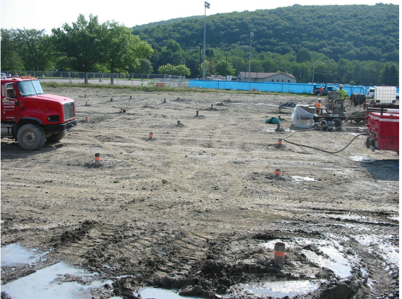
Figure 2. Photograph showing grouting of completed bores following installation of closed-loop tubing at the Owego-Apalachin Elementary School geothermal field, Tioga County, New York. Photograph by William M. Kappel, U.S. Geological Survey.
