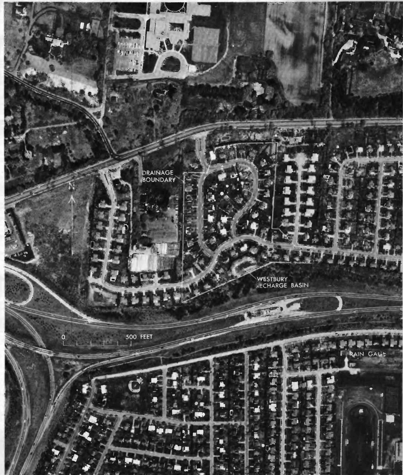
FIGURE 4.—Aerial photograph of the Westbury recharge basin and its drainage area. Photograph by Lockwood, Kessler, and Bartlett.
