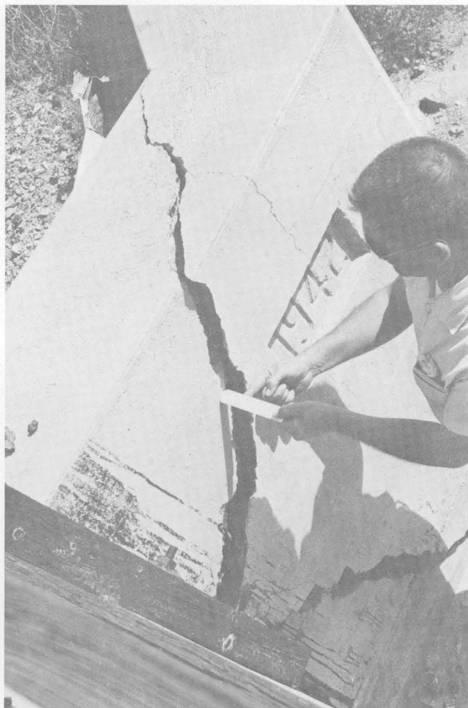
FIGURE 128.—Cracked concrete railroad bridge abutment about 0.3 km southeast of Glamis. Gaping cracks shown here reportedly widened at the time of the earthquake from \frac{1}{2} - to 1-cm openings to 8–10 cm.
