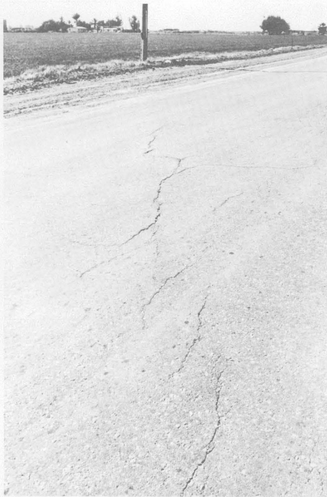
FIGURE 57. — En echelon cracks on Meloland Road first observed following the Imperial earthquake of 1966 (Brune and Allen, 1967a) but slightly widened during the Borrego Mountain earthquake. Fault displacement of about one-half m occurred at this same locality in 1940. Photograph taken April 28, 1968.
