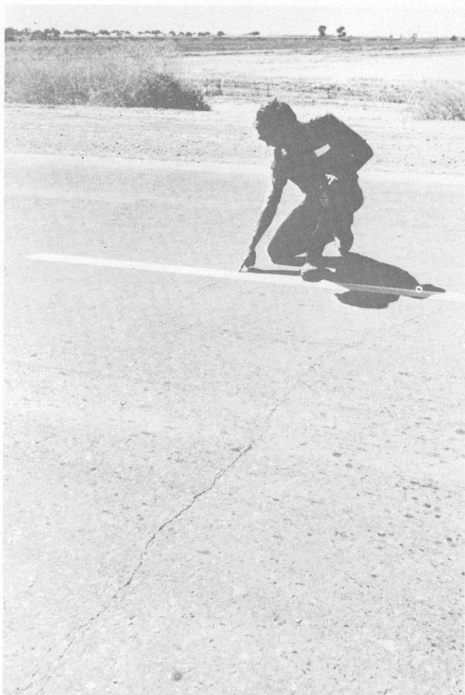
FIGURE 58. — Fresh cracks across Heber Road. Displacement of about 1\frac{1}{2} m took place here in 1940, but no further displacements are known to have occurred here until 1968. Photograph taken April 28, 1968.
