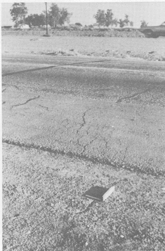
FIGURE 53.—Fresh cracks in unconsolidated material (beneath ruler) at north edge of Highway 80. Older tar-filled cracks in pavement resulted from earlier movements at this locality. (See Brune and Allen, 1967a.) Photograph by R. D. Nason, April 13, 1968.
