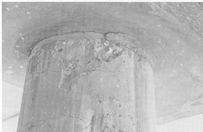
FIGURE 127.—Cracked and spalled 40-cm-diameter concrete pier supporting the Highway 78 bridge over San Felipe Creek, about 8 km east of Ocotillo Wells.
