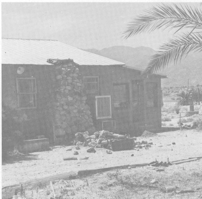
FIGURE 122.—Partly toppled fieldstone chimney in community of Ocotillo Wells.
