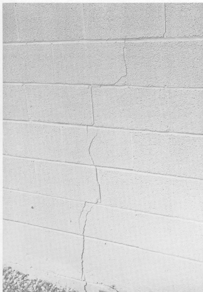
FIGURE 125.—Cracked reinforced concrete-block wall in Salton City building.
