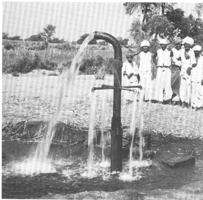
FIGURE 42.—Artesian well drilled by the Government of Saurashtra for the village water supply of Sushiya. Well taps confined sand aquifer in Pliocene deposits at a depth of about 137 m.
