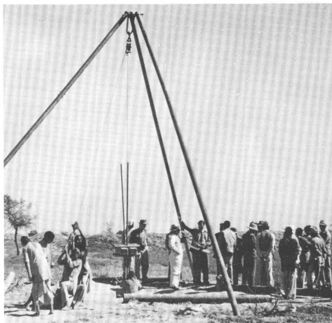
FIGURE 39.—Drilling of irrigation well by tripod and manually operated drill stem and bailer in the Ganges Plain of Uttar Pradesh.
