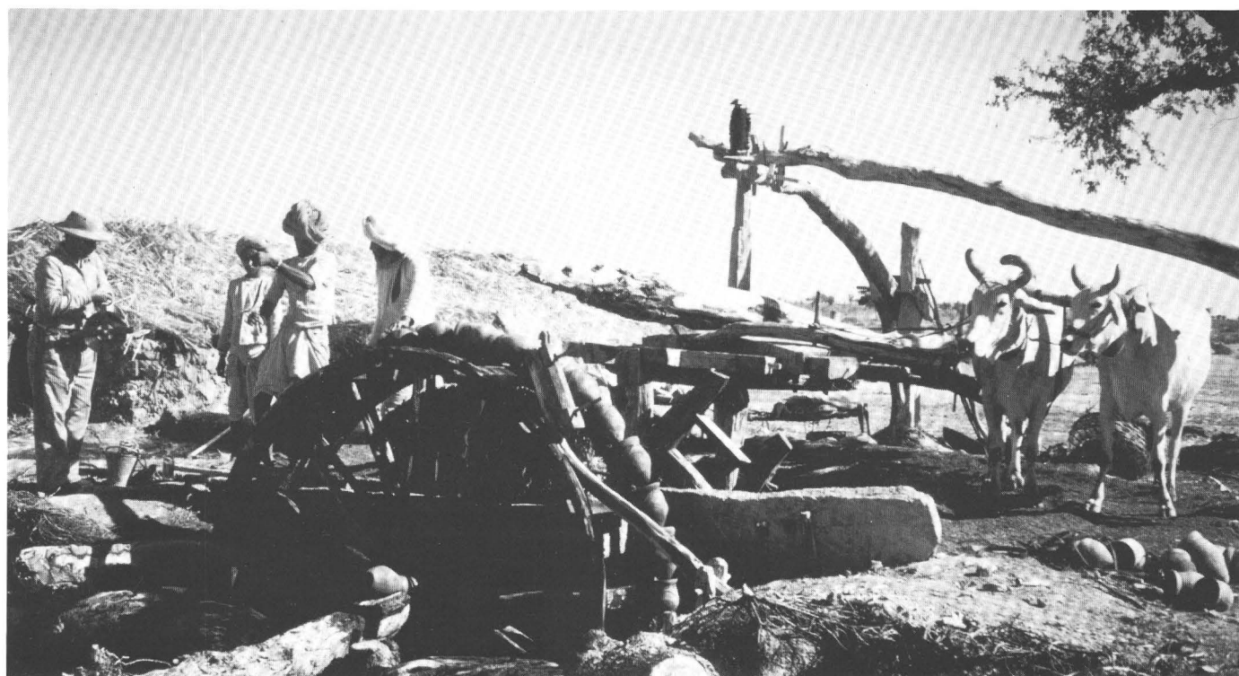
FIGURE 41.—Indian hydrogeologist of the Geological Survey of India measuring water level in dug well near Bhawi in Rājasthān. Well is equipped with Persian water wheel driven by bullocks and taps ground water in Precambrian Aravalli slate.
