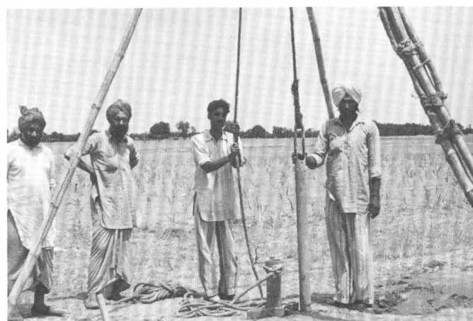
FIGURE 40.—Indian drillers constructing 15.2-cm drilled well using bamboo tripod and hand-powered bailer in Hoshiarpur area, Punjab (Haryana).
