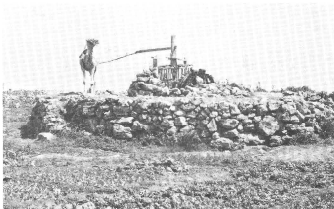
FIGURE 25.—Camel-driven water-wheel or “noria” used to recover ground water from shallow dug well in semiconsolidated deposits of dune sand and coquina. Such wells are used to irrigate small vegetable gardens along the Atlantic Coast between El Jadida and Safi.
