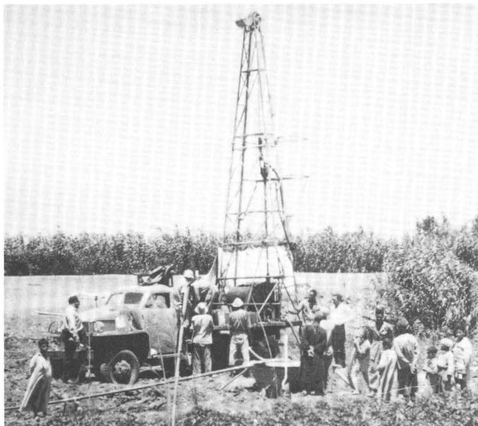
FIGURE 12.—Drilling of observation well by light rotary rig in the Nile Delta south of Ziftá.
