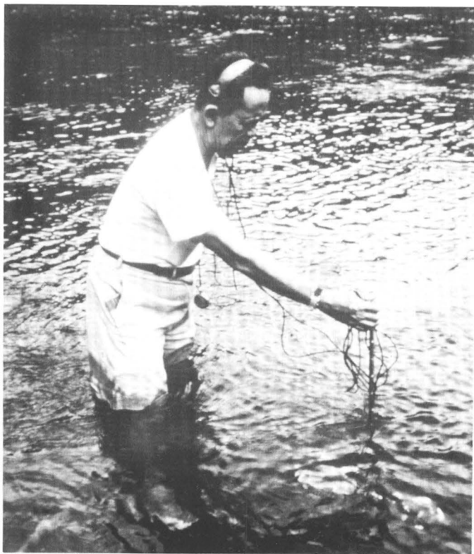
FIGURE 54.—Philippine hydrologist of the Hydrographic Section, Bureau of Public Works making current-meter measurement on Angat River in Luzon.
