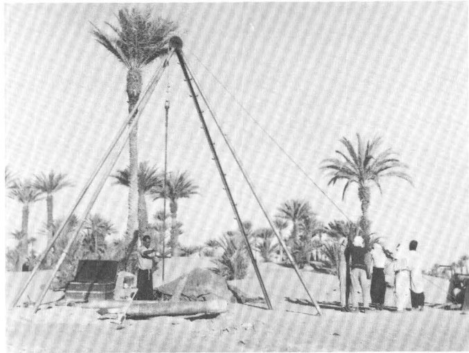
FIGURE 21.—Libyan technicians operating hand-powered drilling rig in the Wādī ash Shātī under direction of USGS hydrogeologist, G. C. Tibbitts, Jr. Driller at left turns drilling rod to rotate bit. Men pull down on drilling line, lifting bit, which drops about 45 cm on release of line. Hand winch at right raises and lowers tools.
