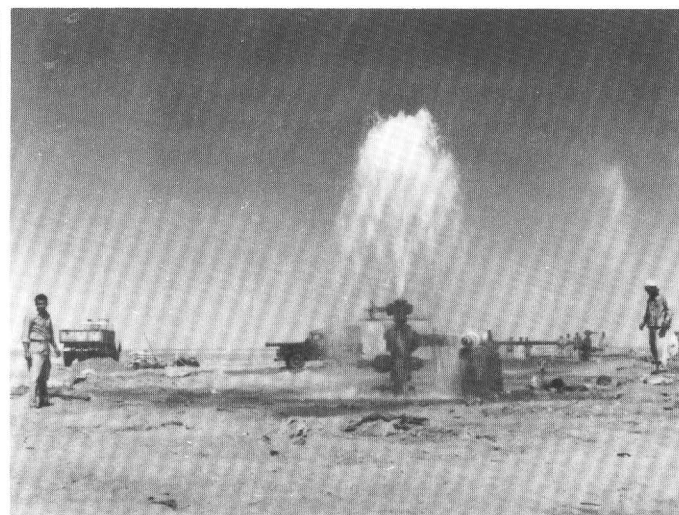
FIGURE 16.—Two flowing artesian wells put down in Al Wāhāt al Kharijāh as part of the New Valley pilot ground-water development project. Nasser no. 3 at the left is 650 m deep and flowed initially 5,100 m 3 per day; Nasser no. 1 at the right is 400 m deep and flowed initially 8,000 m 3 a day. Both wells tap sandstone aquifers in the Nubian Series.
