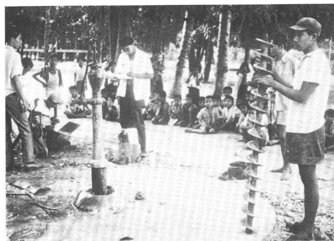
FIGURE 56.—Thai engineers and geologists recording observations during installation of hand pump on recently drilled well at Nong Tuloom school, 6 km south of Nakhon Ratchasima (Khorat). School children in background are interested observers.
