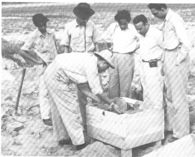
FIGURE 43.—Indian hydrogeologists of the Geological Survey of India installing automatic water-stage recorder on observation well in West Bengal.
