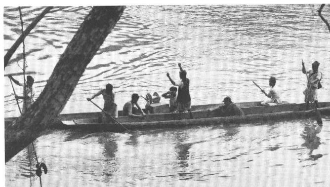
FIGURE 47.—Nepalese technicians stringing cable from two dug-out canoes for gaging station on the Karnālī River at Chisāpani.
