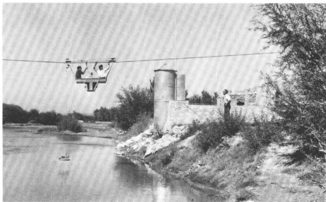
FIGURE 38.—A. O. Westfall, USGS hydrologist, instructing Afghan hydrometrists in stream-gaging methods by cableway at model gaging station on Kābul River near head of Tang-e Ghārū. View upstream.
