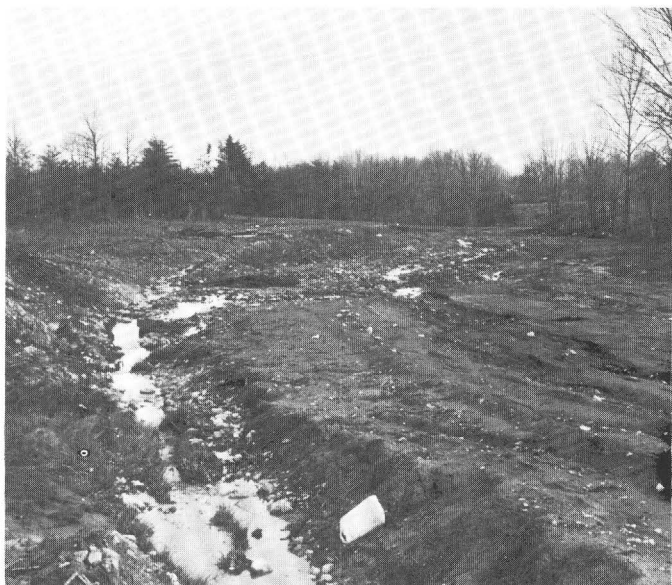
FIGURE 21.—Grading for street right-of-way within the Manor Run stream channel, 1967.
