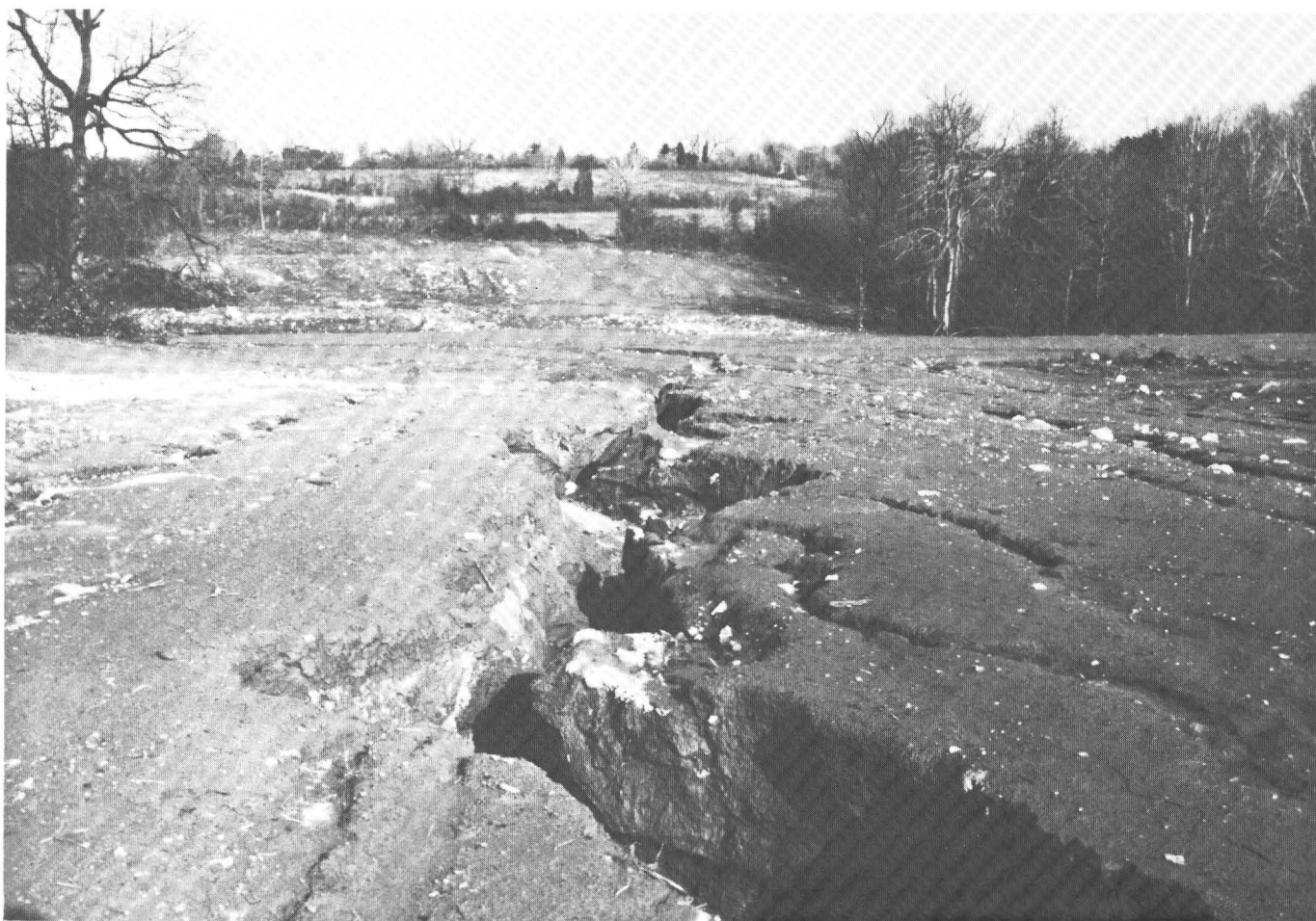
FIGURE 17.—Extensive erosion in the Manor Run basin, 1967.
