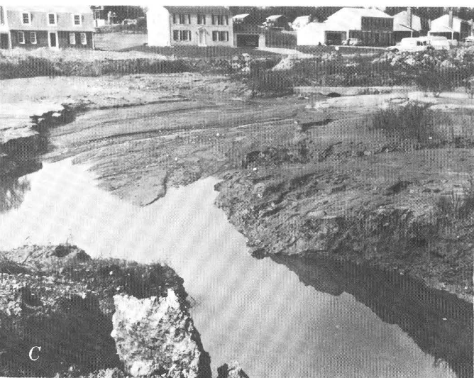
FIGURE 26.—Sediment basin before (A) and after (B and C) it was breached for installation of a sewer line. Note the scour of previously accumulated sediments.
