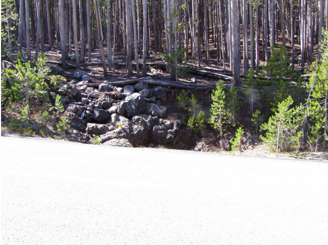
Looking south across highway at bench mark (beneath yellow case).
