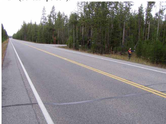
Looking west along highway at T-junction and person (pointing at bench mark).
