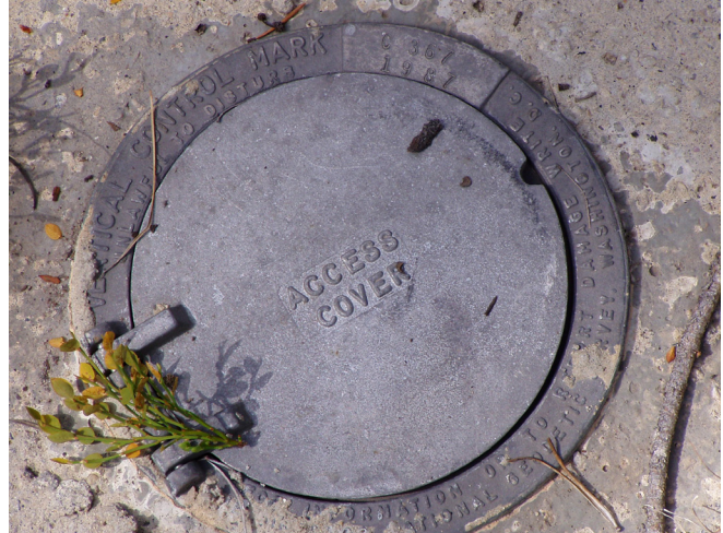
Close up of bench mark.
