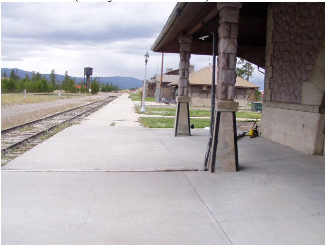
Looking west along the south side of the building at bench mark (near yellow GPS unit).
