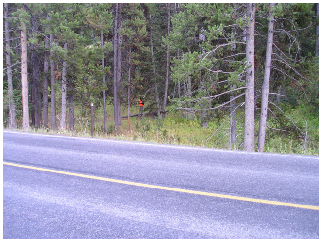
Looking south across highway at culvert marker (brown post with white reflector on top) and bench mark (beneath person).
