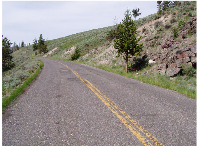
Looking north along highway at bench mark (beneath orange marker).
