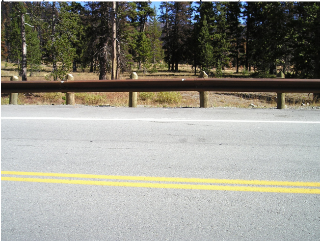
Looking north from Cub Creek Bridge at bench mark (near orange dot in the distance).
