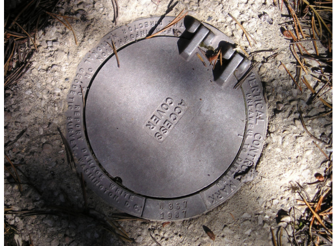
Close up of bench mark.
