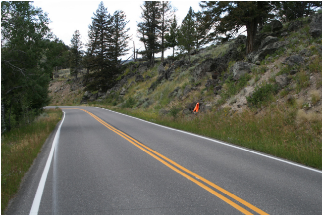
View west along highway at bench mark (near orange vest).
