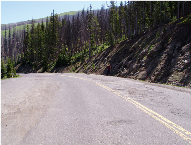
Looking north along highway at bench mark (beneath yellow GPS datalogger).
