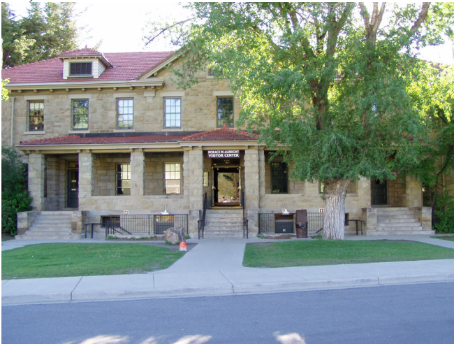
Looking north at the visitor center and bench mark (under orange hard hat).
