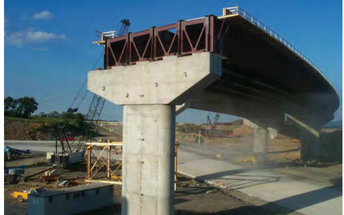
Figure 8. Overpass under construction, near State College, Pennsylvania.
