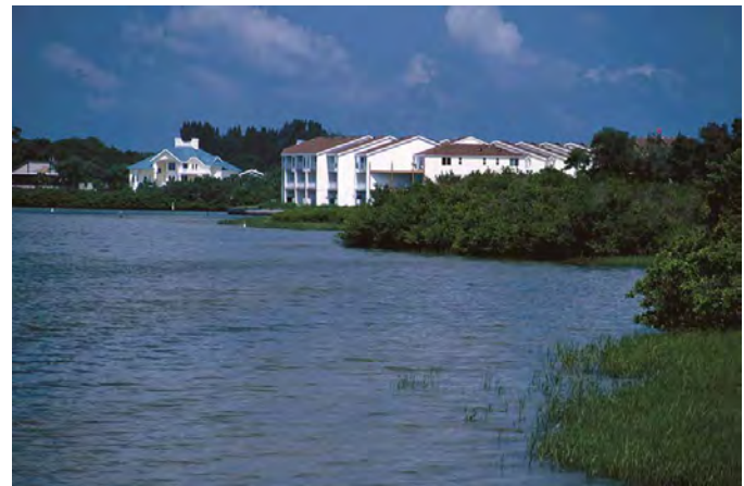
Figure 4. Large waterfront homes and apartment complex, examples of intensive development along Tampa Bay, Florida.
