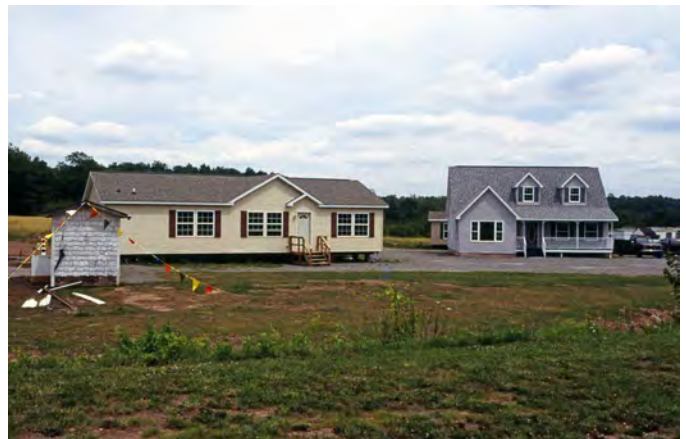
Figure 8. Modular homes waiting to be transferred to housing sites, in North Central Appalachians Ecoregion.
