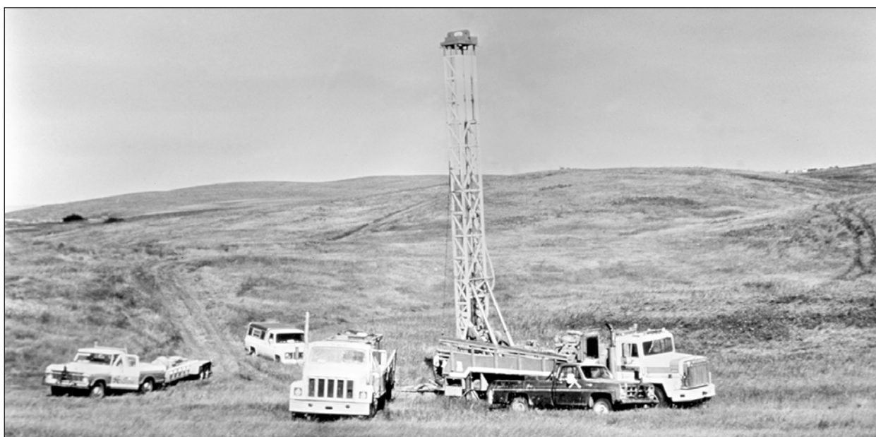
Figure 7. Commercial drill rig installing a groundwater-monitoring well at the Cottonwood Lake study area, North Dakota, 1978. Photograph by U.S. Geological Survey.
